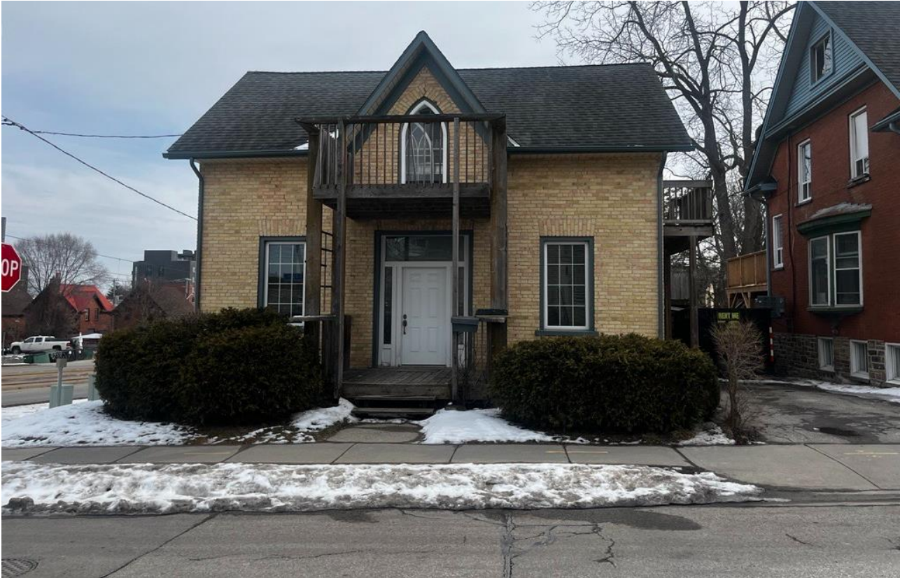
Figure 2: Front Façade of Subject Property
