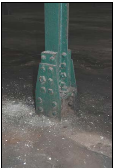
Fig. 32 riveted shear plate column
