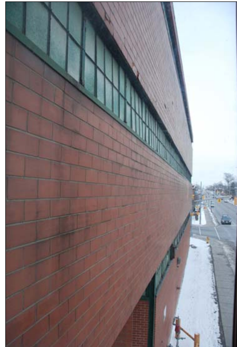
Figure 27 horizontal strip windows
