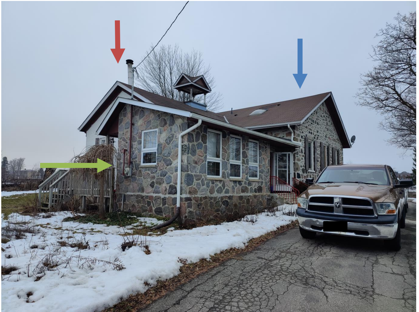
Figure 3. Phases of construction of the Williamsburg Schoolhouse. The blue arrow points to the original schoolhouse built in 1864, the red arrow points to the brick addition added in 1874, and the green arrow points to the stone-faced, wood frame addition added in 1987.
