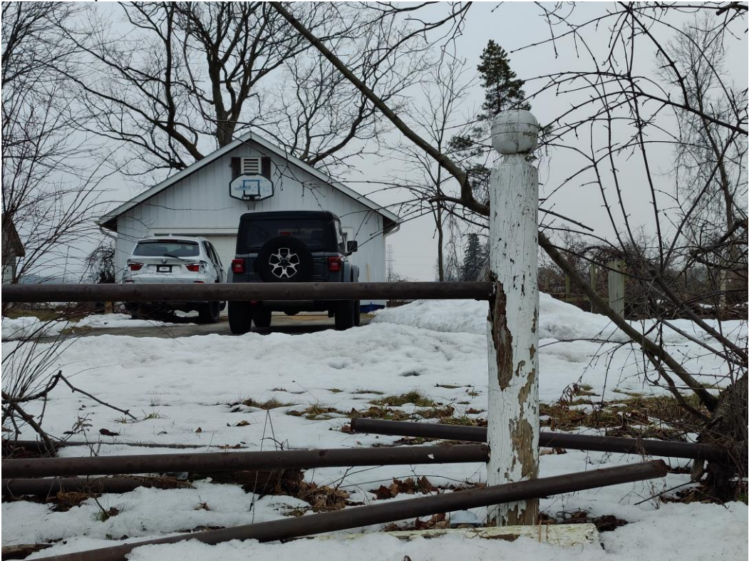
Figure 6. Current condition of the post and rail fence.
