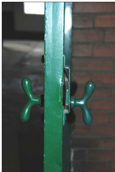
Fig. 33 door hardware at stairwell
