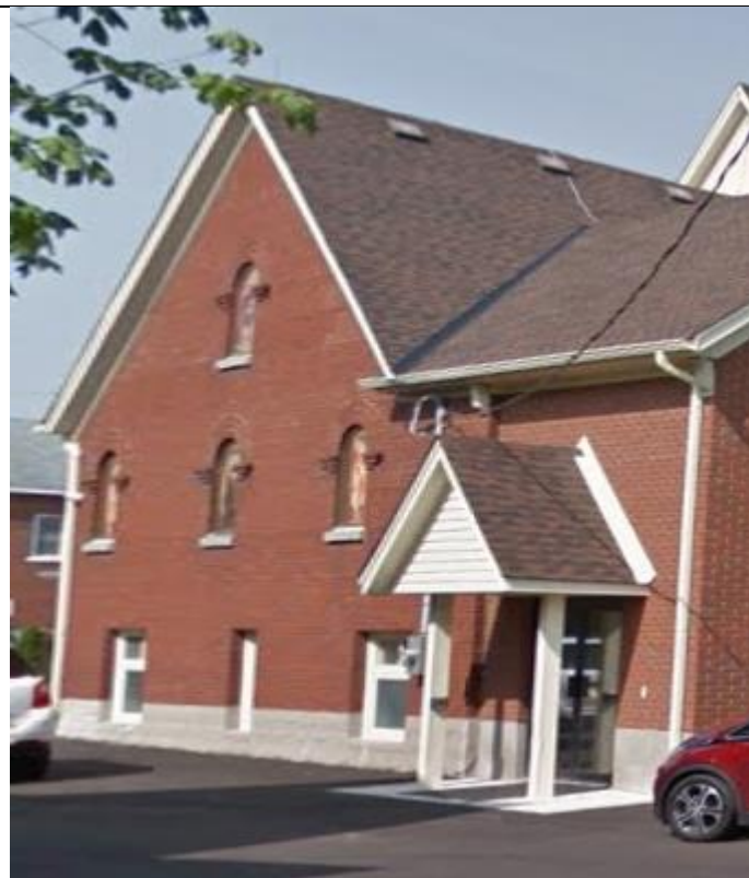
Rear Elevation (East Façade)
