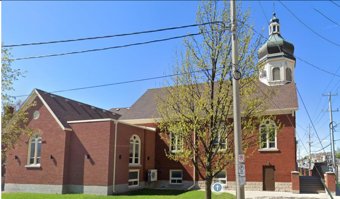
Side Elevation (North Façade)
