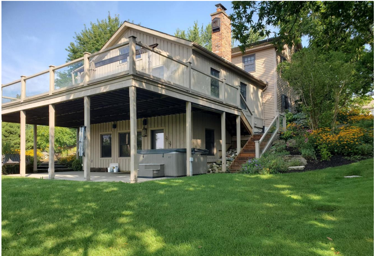
Figure 3: Existing Rear Deck and Patio
