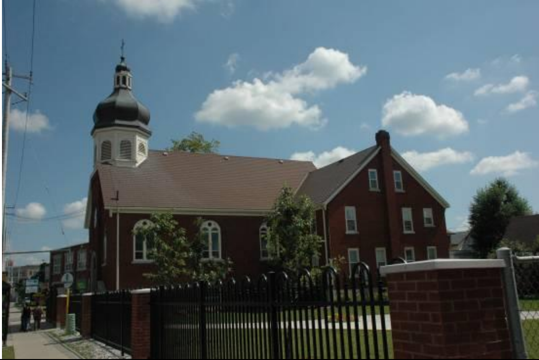
Side Elevation (South Façade)
