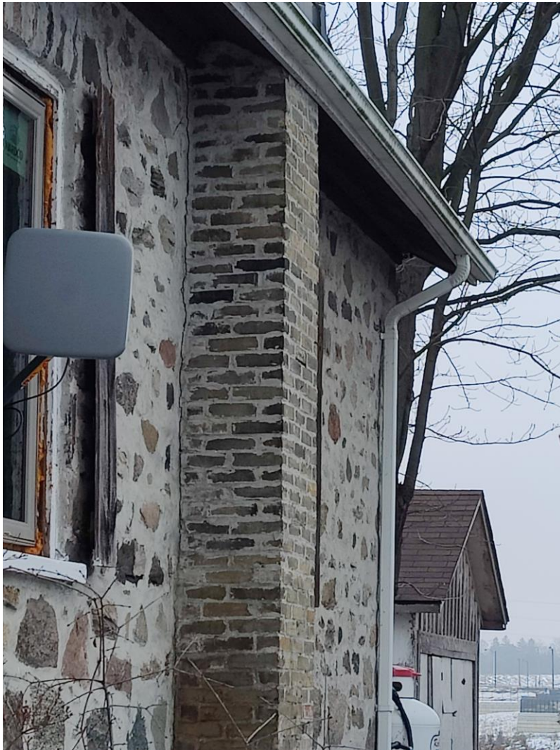
Figure 5. Current condition of the chimney
