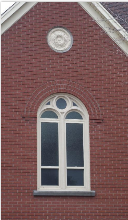
Photograph showing the details on the north 2015 building addition
