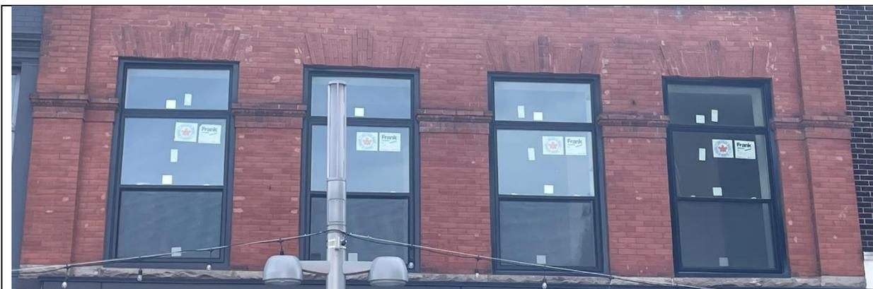
Detailing of second-storey showing flat head window openings; rectangular transoms; 1/1 windows; and, brick voussoirs and continuous stone sills
