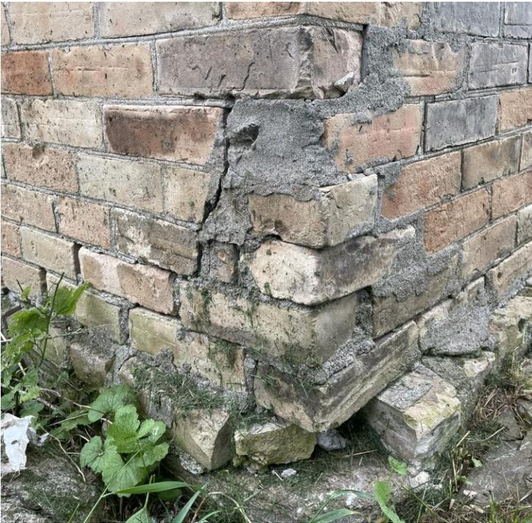
**Figure 5.0: Photograph showing missing bricks, step cracks and inappropriate mortar repairs**
