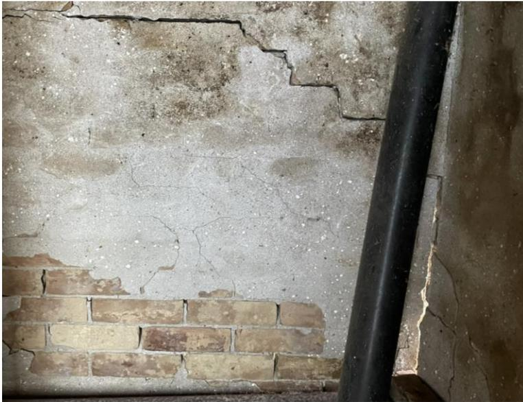
**Figure 3.0: Photograph showing major cracks through the parging and mortar where you can see through the smoke house**
