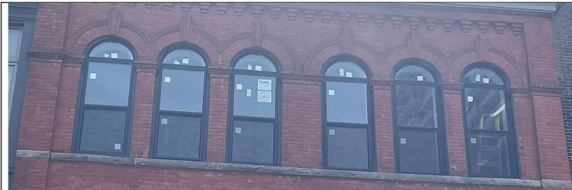
Detailing of second-storey showing semi-circular window openings; semi-circular transoms; 1/1 hung windows; and, decorative brick hood moulds with keystones and continuous stone sills
