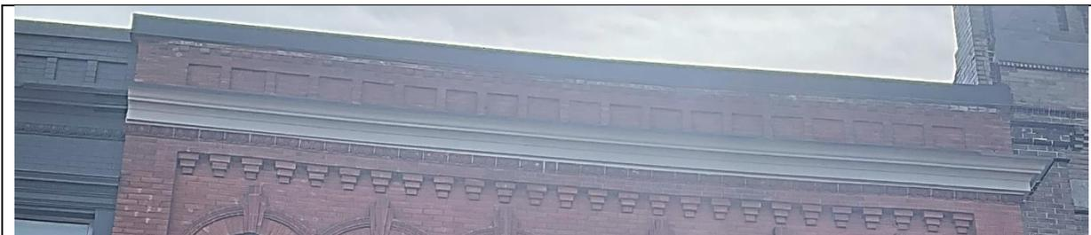
Detailing of brick frieze, stone and brick architrave and ornamental brick moulding along with red brick corbelling – 97-99 King Street West
