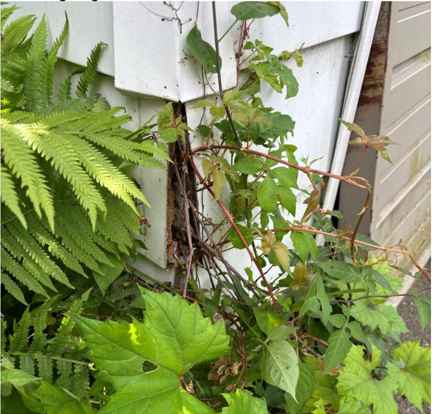
**Figure 5:** Branches protruding from the corner of the garage
