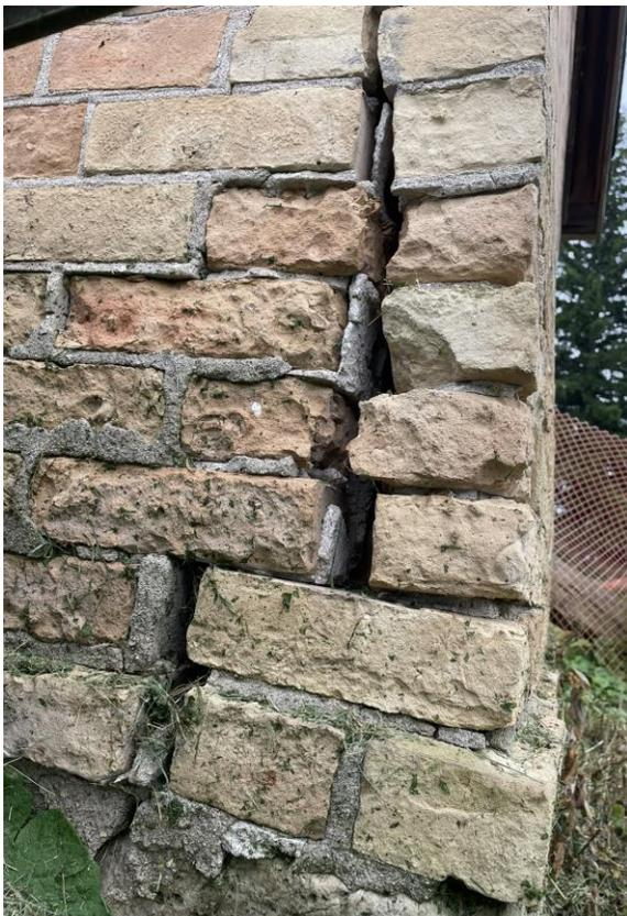
**Figure 7.0: Photograph showing shifted foundation**
