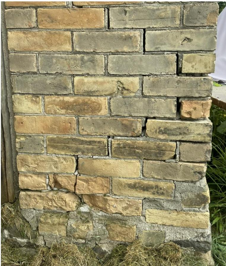
**Figure 4.0: Photograph showing step crack and spalling bricks**
