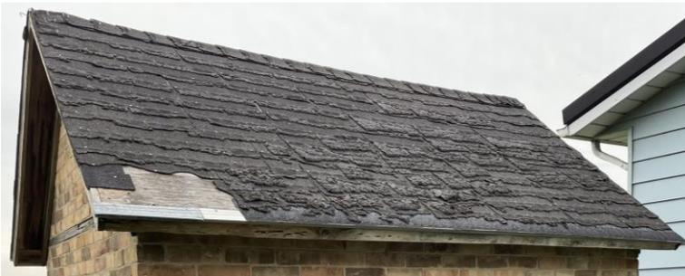
**Figure 6.0: Photograph showing deteriorated/missing asphalt shingles**
