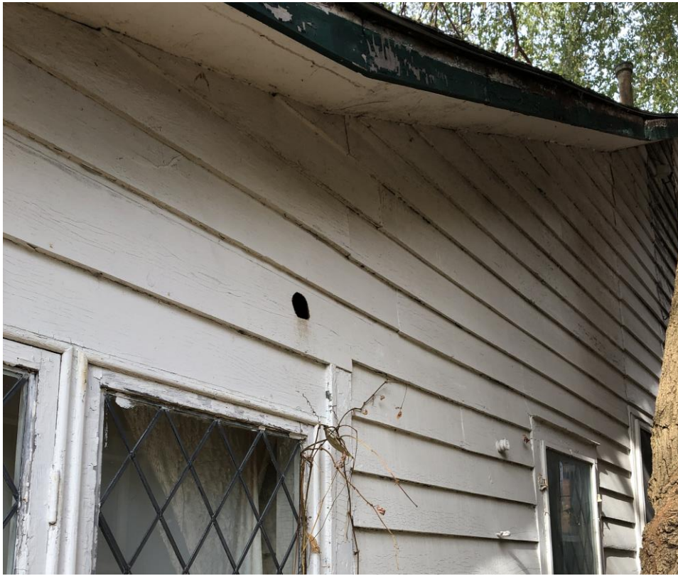
Photo 3. Side (East) Elevation in 2023
