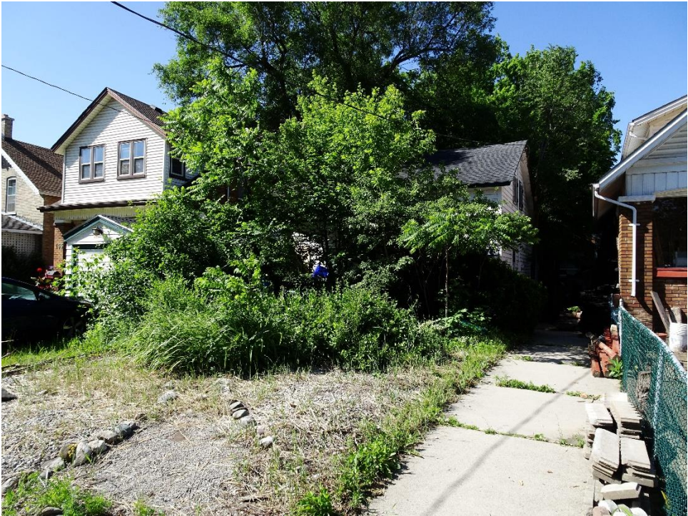
Photo 1. Front (North) Elevation in 2020
