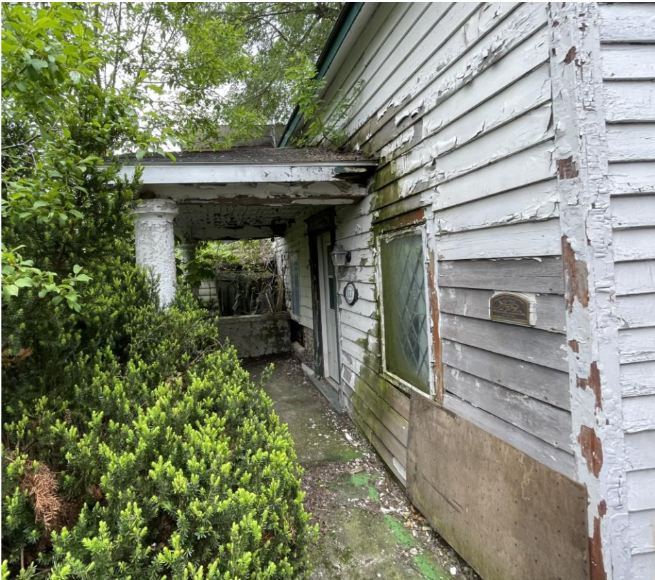
Photo 5. Front (North) Elevation in 2024
