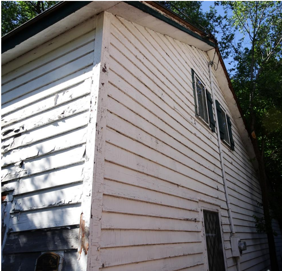
Photo 4. Side (West) Elevation in 2020
