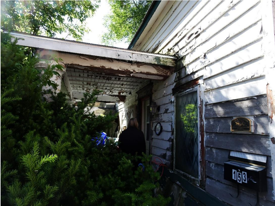
Photo 2. Front (North) Elevation in 2020
