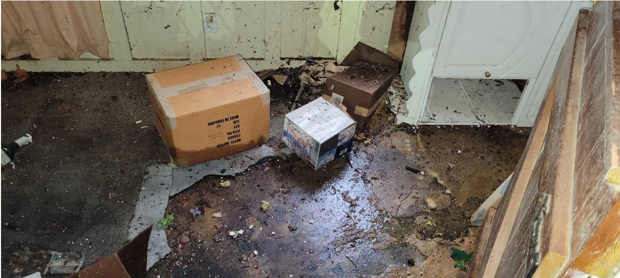
Figure 15. Interior – Floor in 2023
