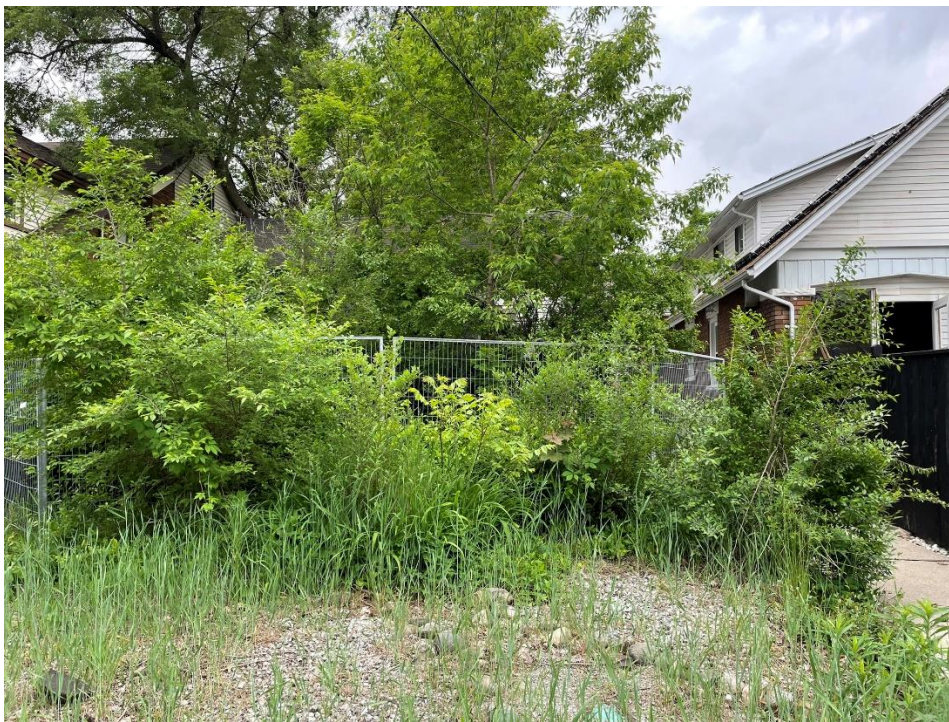
Figure 19. Front (North) Elevation in 2024
