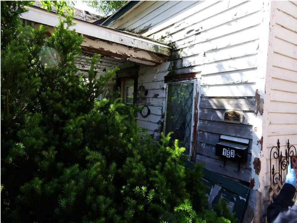
Photo 1. Front (North) Elevation in 2020
