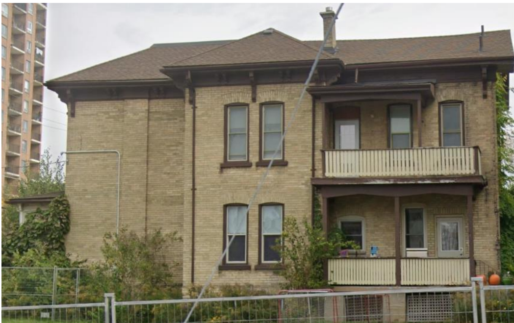
Side Elevation (West Façade) – 83 Benton Street
