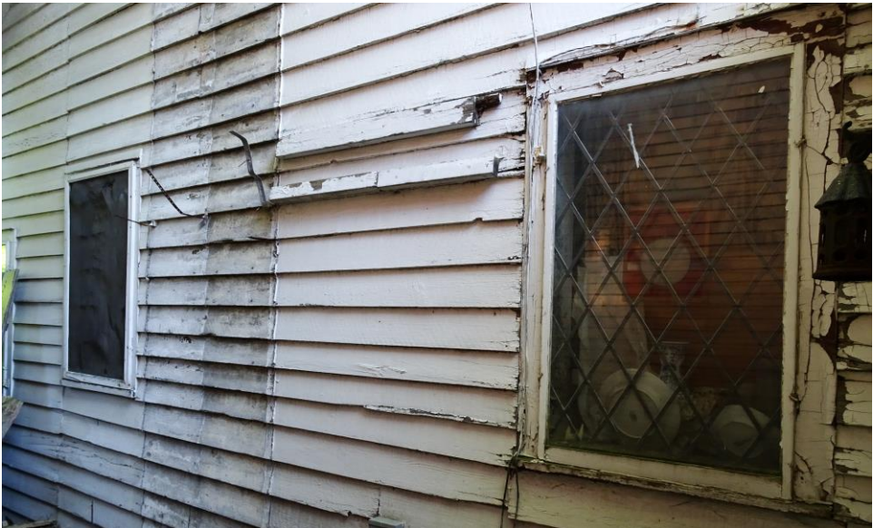
Photo 2. Side (East) Elevation in 2020
