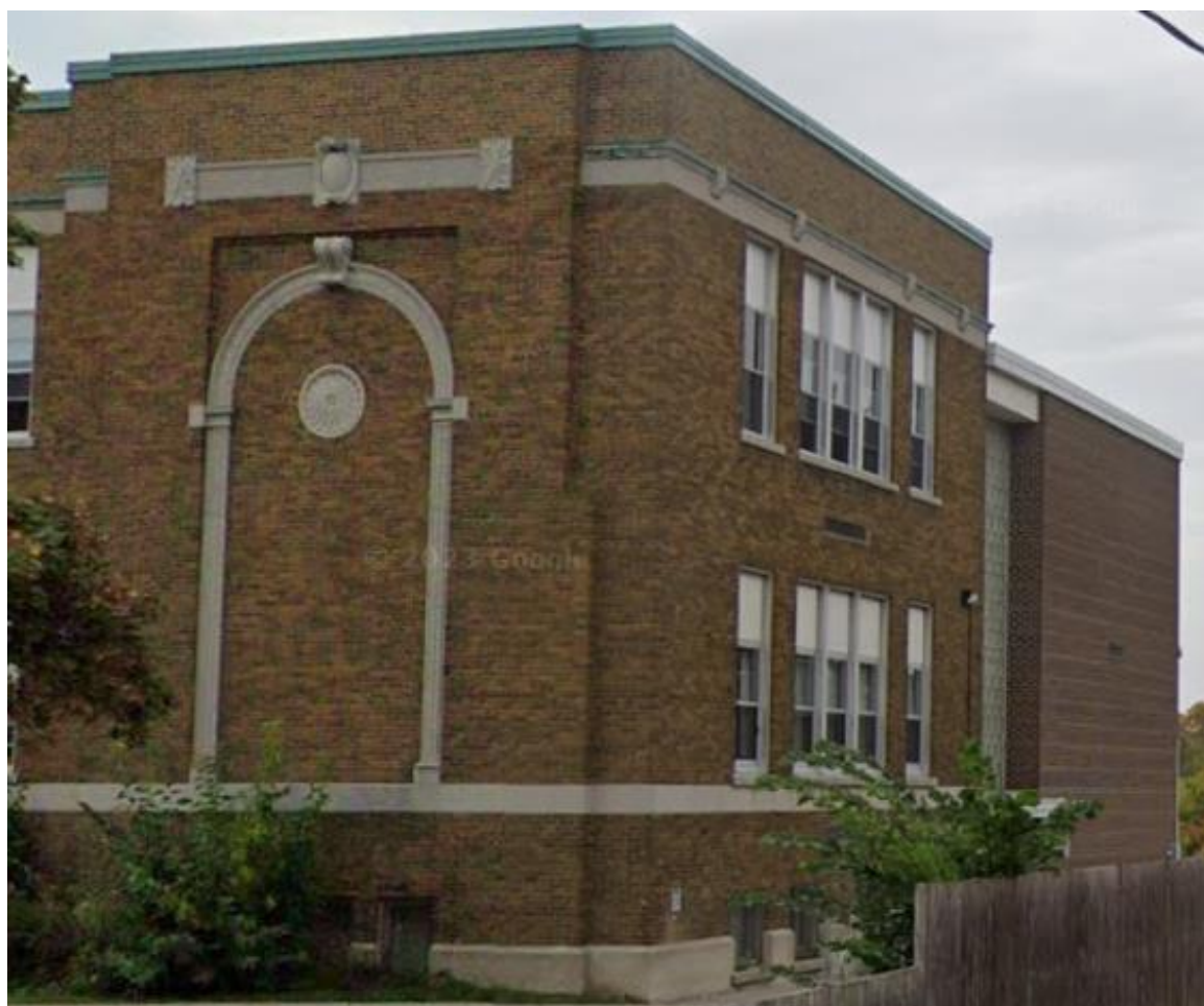
Side Elevation (West Façade) – 107 Courtland Avenue East
