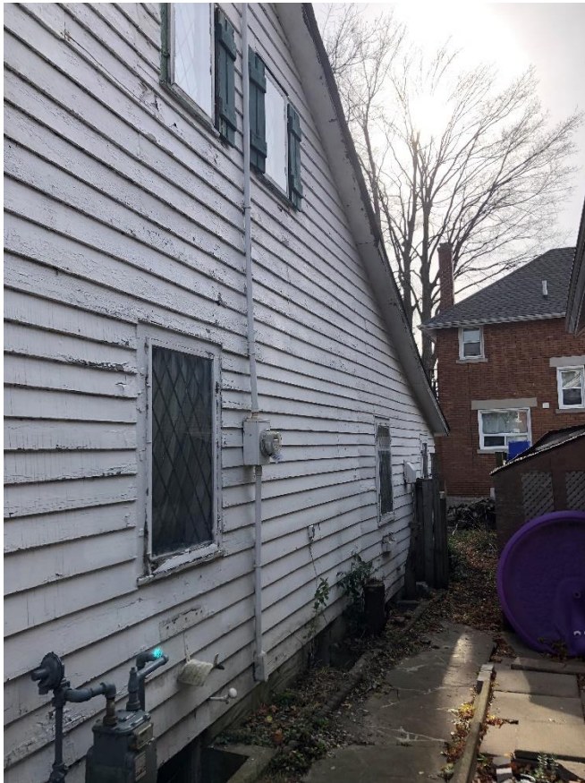
Figure 8. Side (West) Elevation in 2023
