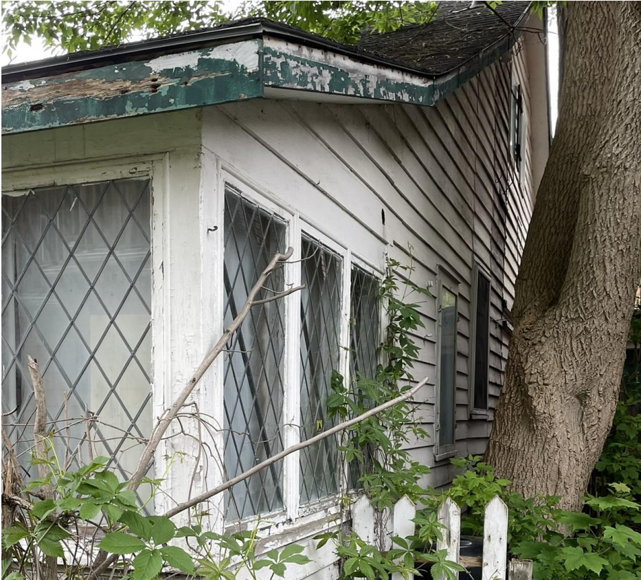
Photo 6. Side (East) Elevation in 2024
