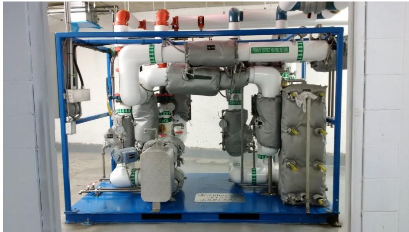
Figure 26: Space Heating and DHW ETS Skid 7
