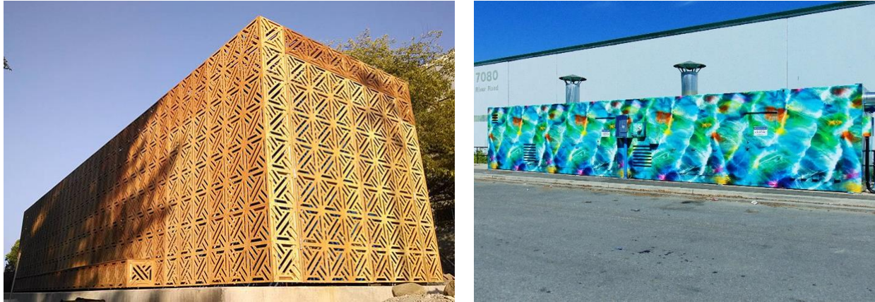
Figure 29: Interim Energy Centres at UBC (left) 9 and Oval Village (right) 10
