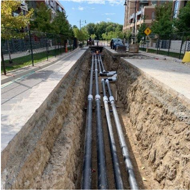
Figure 4: Example of a Distribution Piping System
