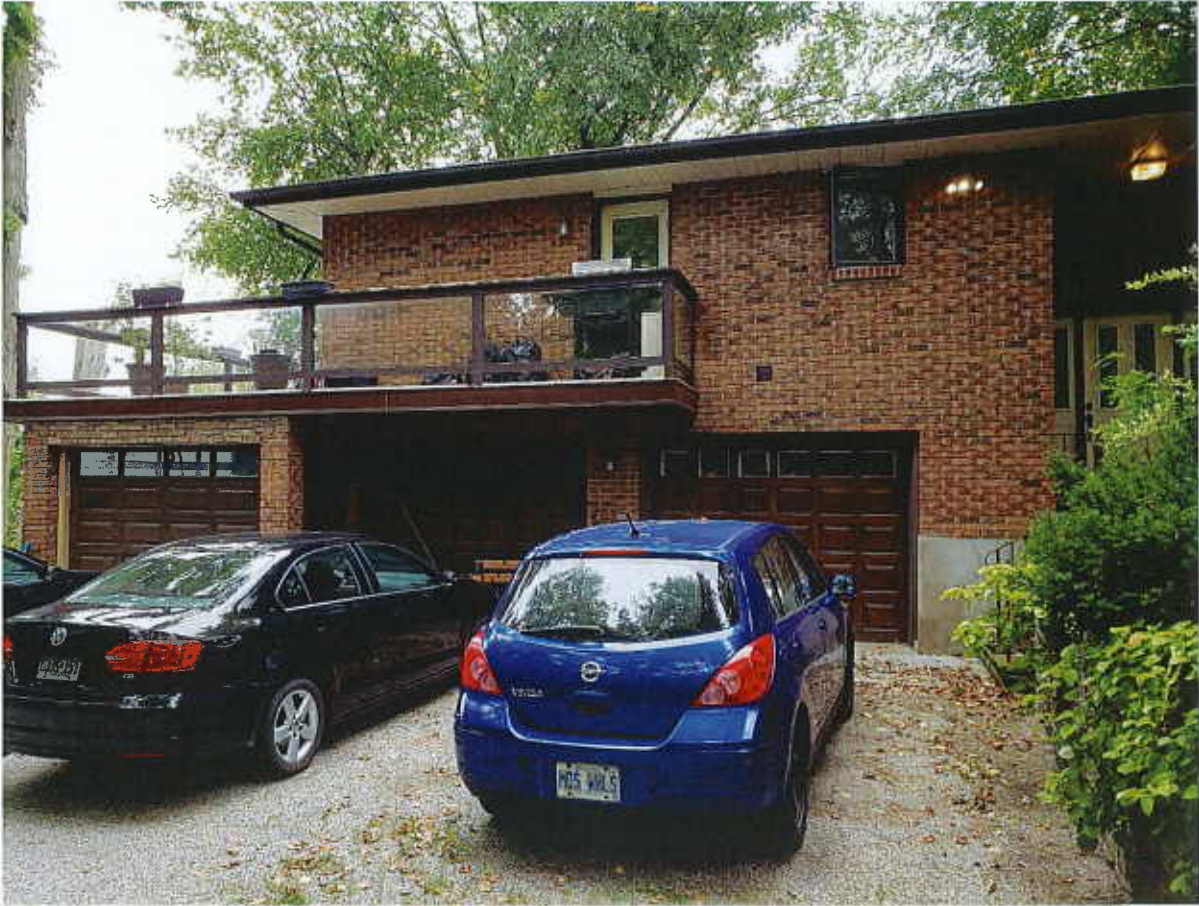
Additional view of the front side of our house showing full Eastern extent of house and porch
