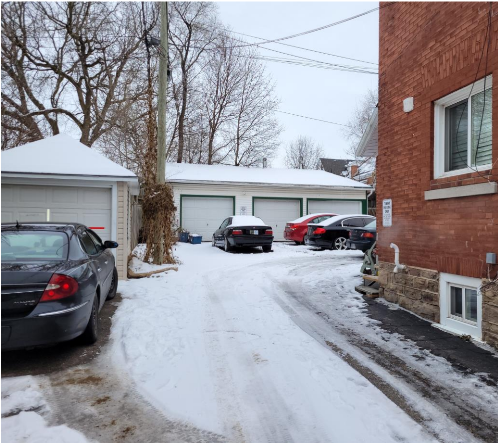
Figure 3 - Metal-clad garage at rear of property
