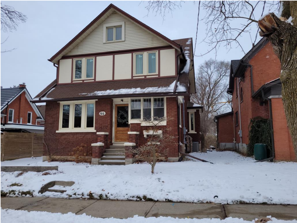
Figure 4 - Photo of 44 Betzner Avenue North
