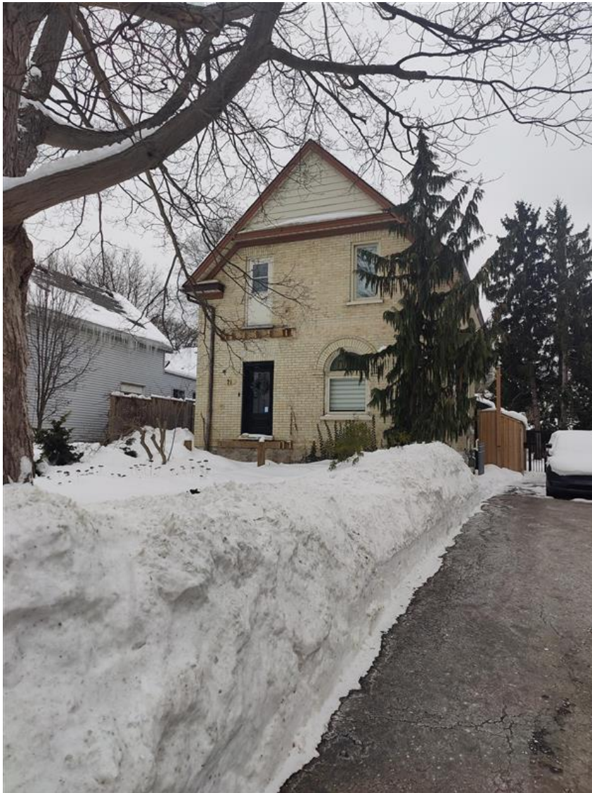
Figure 3. Current Condition of the front porch.
