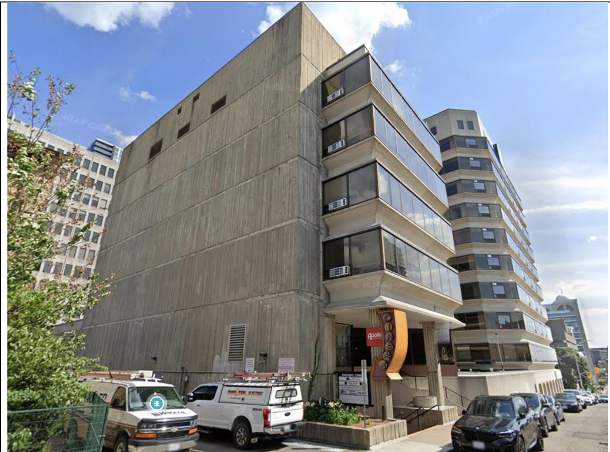
Rear Elevation (North Façade) (Google, 2024)
