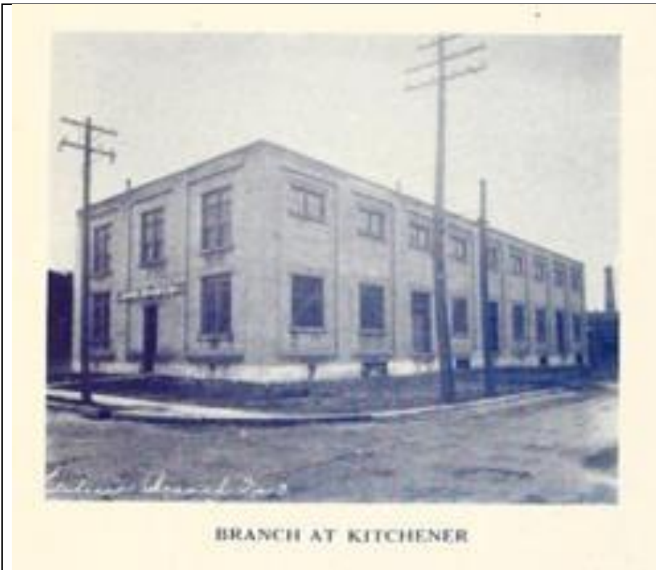
241-247 Duke Street West / 55 Victoria Street North (Canadian Grocer, April-June 1920)
