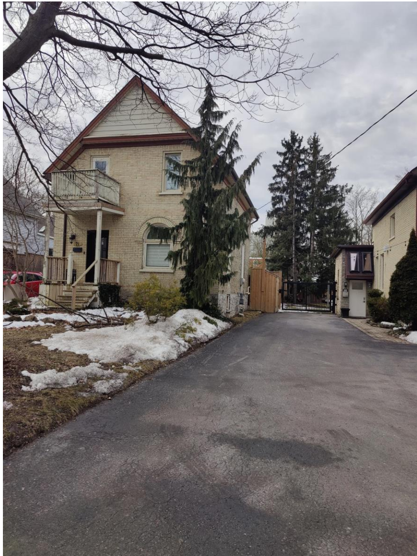
Figure 2. Front Façade of the subject property in 2023
