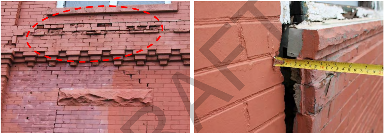
Figures 42 & 43: (left) Secondary view of broken and deteriorated masonry at exterior of Building 1, (right) View of cracks in masonry wall at exterior of Building 2, (MHBC, 2024)
