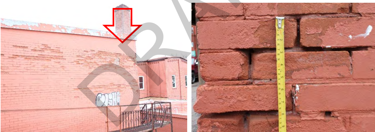
Figures 38 & 39: (left) View of spalling bricks at exterior of Building 1, (right) View of deteriorated masonry at exterior of Building 1 (MHBC, 2024)
