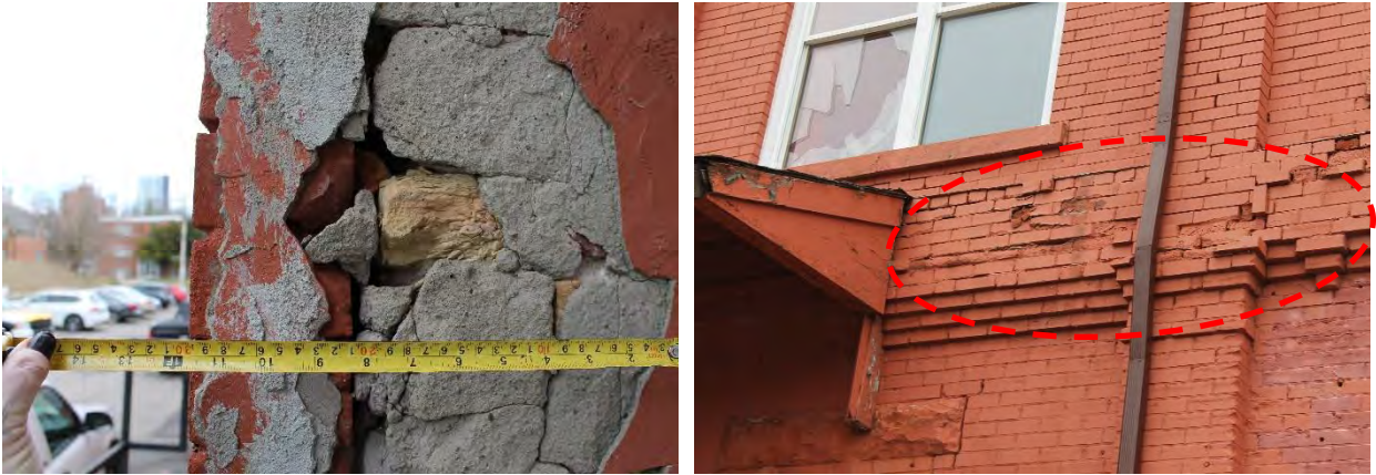
Figures 40 & 41: (left) View of poor masonry repairs at exterior of building 1, (right) View of deteriorated/spalled masonry at exterior of Building 1 (MHBC, 2024)
