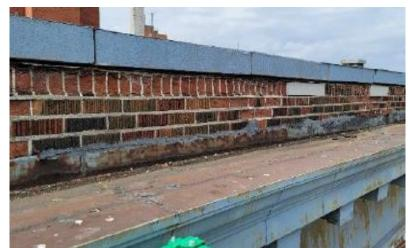
Figure 6: Original Cornice/Parapet with Deteriorated Brick and Metal
