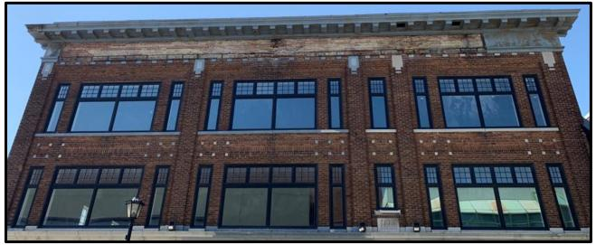
Photo #1: Removed flashing showing exposed brick above
