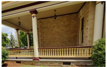
Figure 11: Loose wood-framed porch vents on the side elevation
