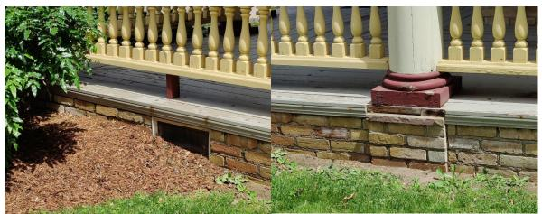
Figure 8: Loose mortar joints in the east (side) elevation
