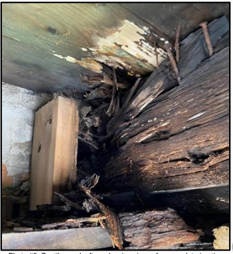
Photo #2: Cantilevered rafters showing signs of severe deterioration
