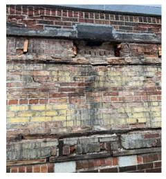
Figure 5: Deteriorated Brick on Wall
