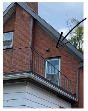
A new window will be replace the existing door. Width to remain to keep brick header detail. Below window, new brick that matches existing will be installed.
