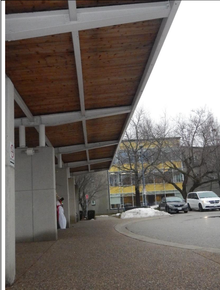
Underside of the canopy has tongue and groove wood.
