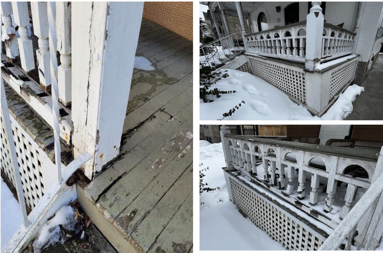
Figures 3-5: Deterioration of Existing Porch
