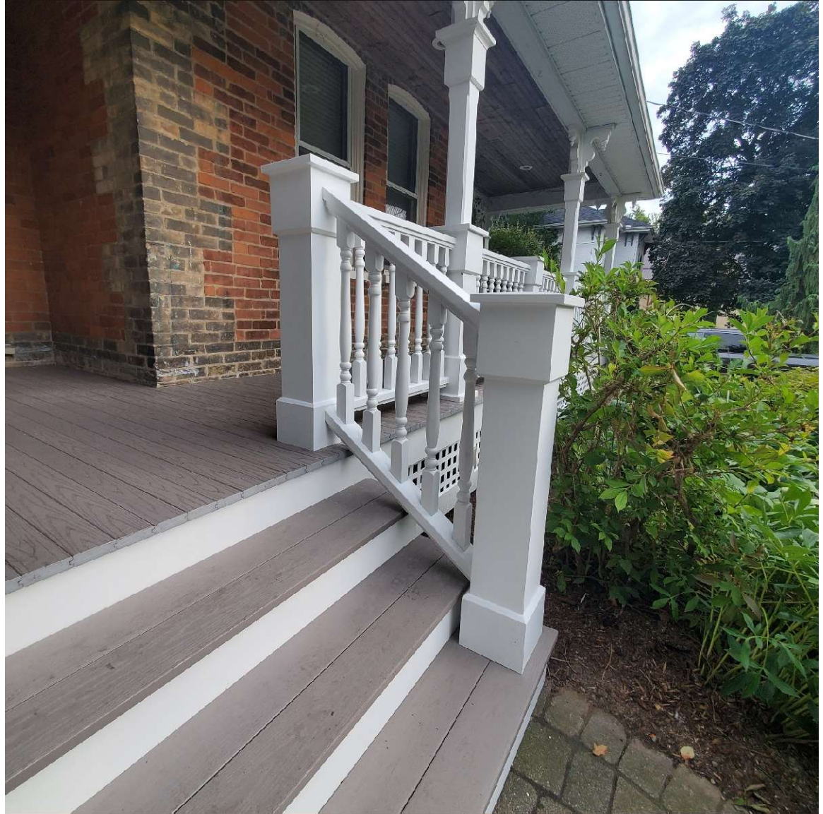
Photo above from a recent project showing Azek slate grey t&g porch plank, Azek 1"x 5 1/2" decking on stair, PVC risers and skirting, and Accoya railing system that was milled to match this particular project.
