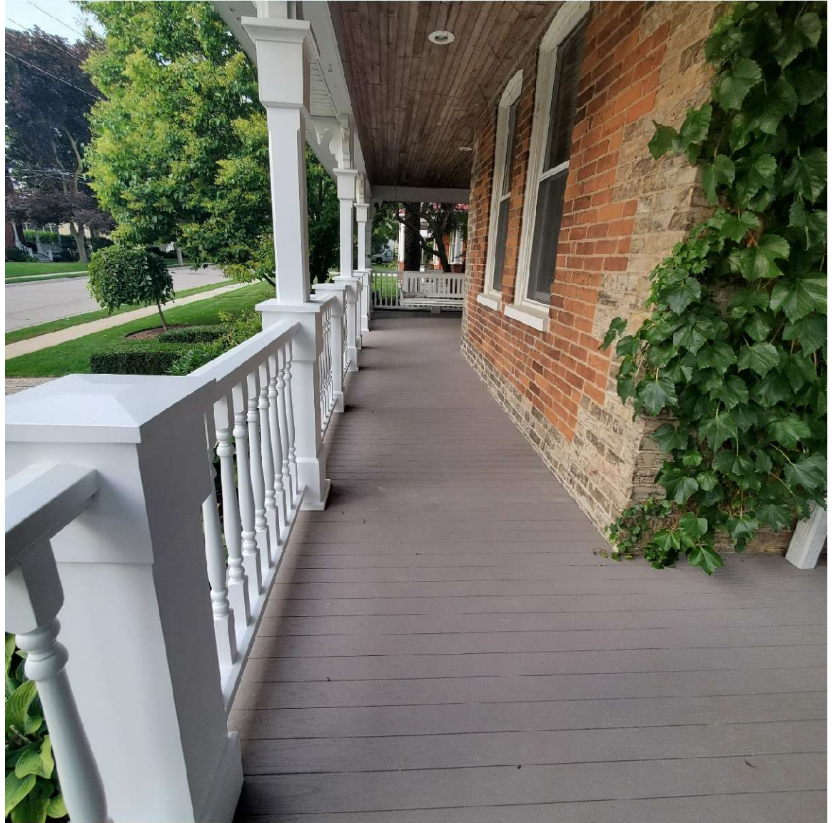
Photo above from a recent project showing Azek slate grey t&g porch plank, and Accoya railing system that was milled to match this particular project.
