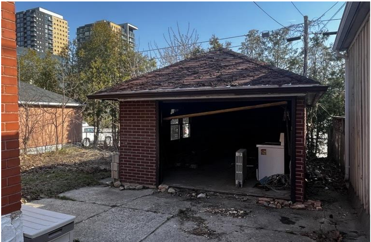
Figure 10: Rear Detached Garage
