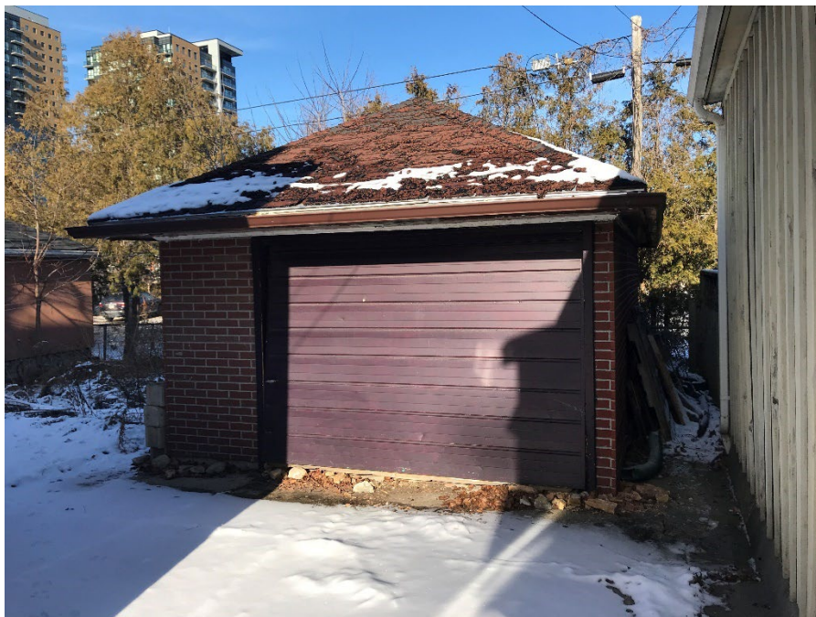
Existing Detached Car Garage
