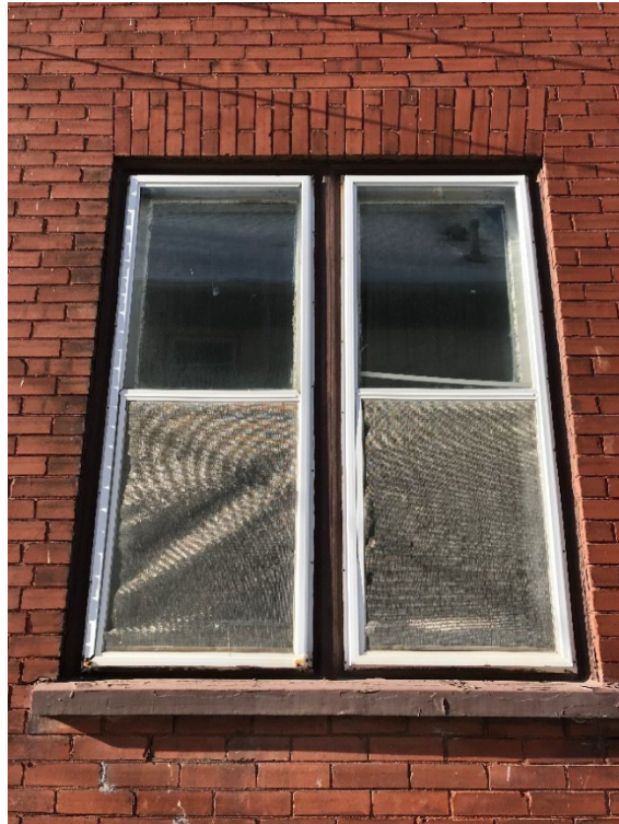
Existing windows & trims.
