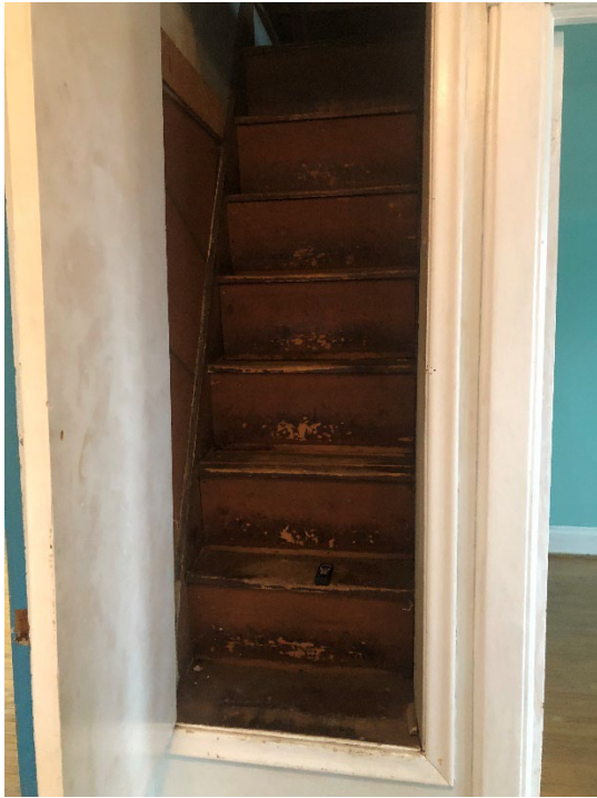
Interior – Relocation & repair of existing stairs to attic.
