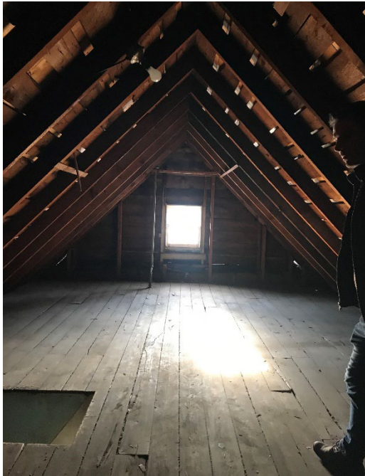
Fig. 01 Photograph of the existing attic.
