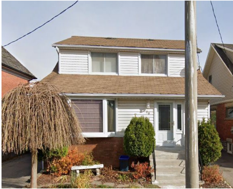
Siding on Dormer.
