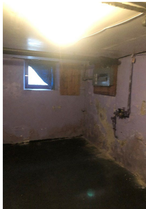
Fig. 06 Photograph of existing basement conditions.
