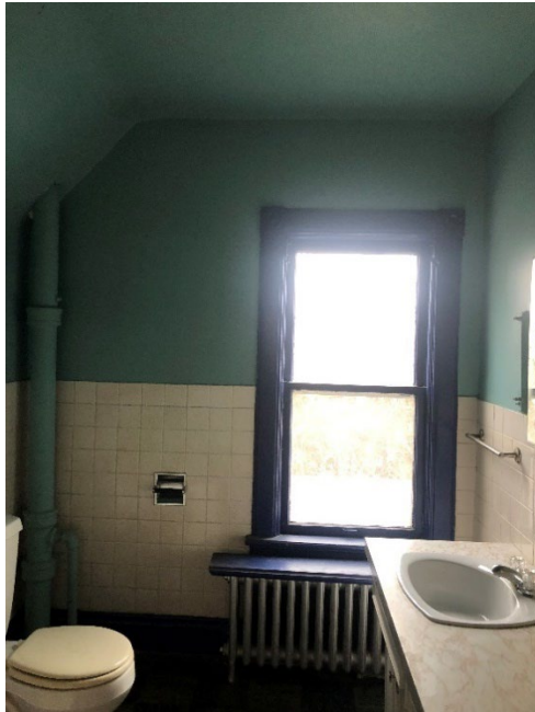
Fig. 10 Photograph of the existing bathroom with an angled ceiling.
