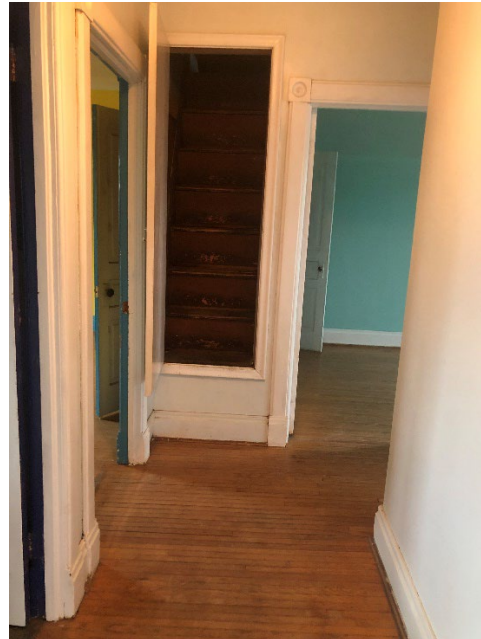
Fig. 04 Photograph of existing stairs to attic.
