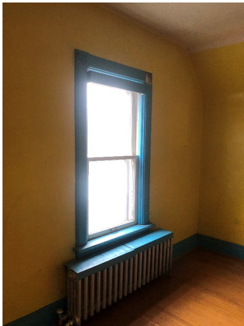
Fig. 11 Photograph of the existing bedroom with an angled ceiling.
