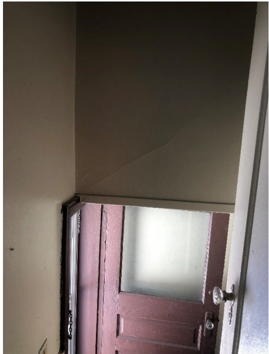
Interior – Propose new headroom clearance. (Exist = 6.5')
