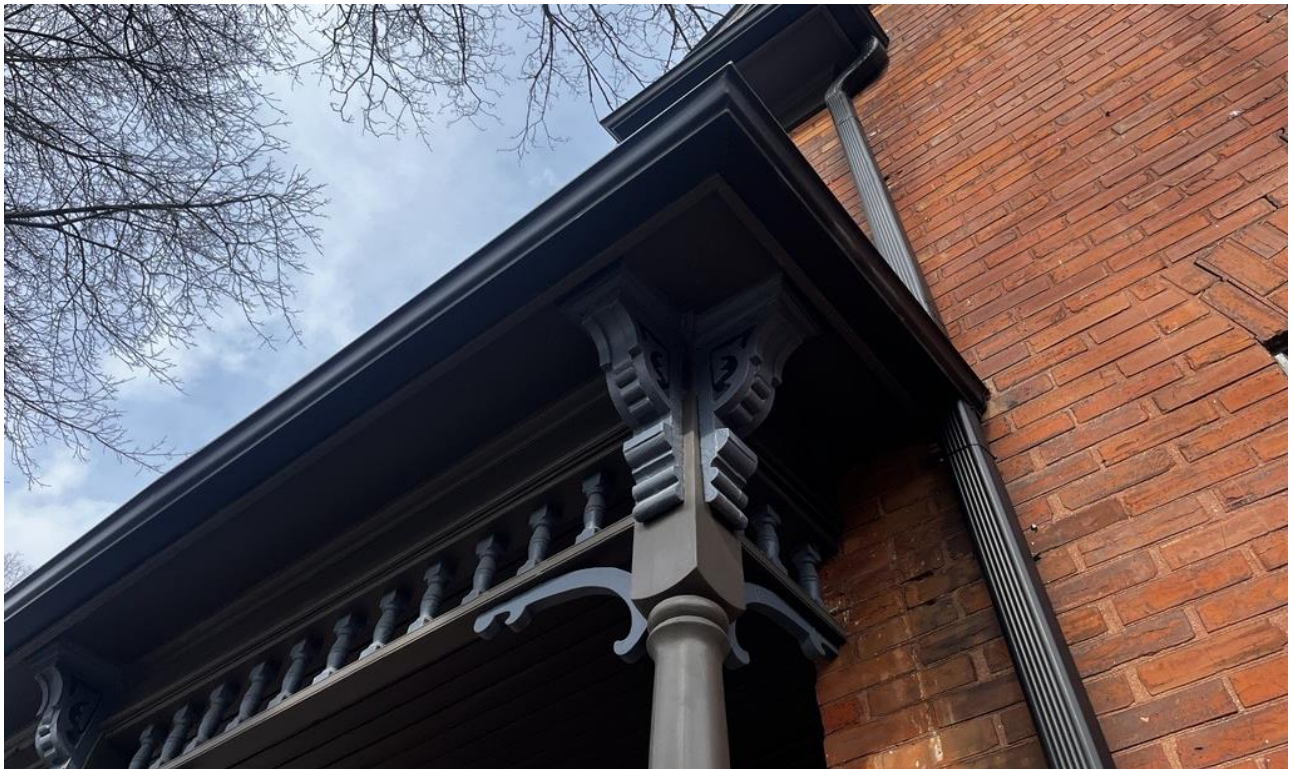
Figure 4: Corner Bracket and Other Detailing on the Wrap-Around Verandah
