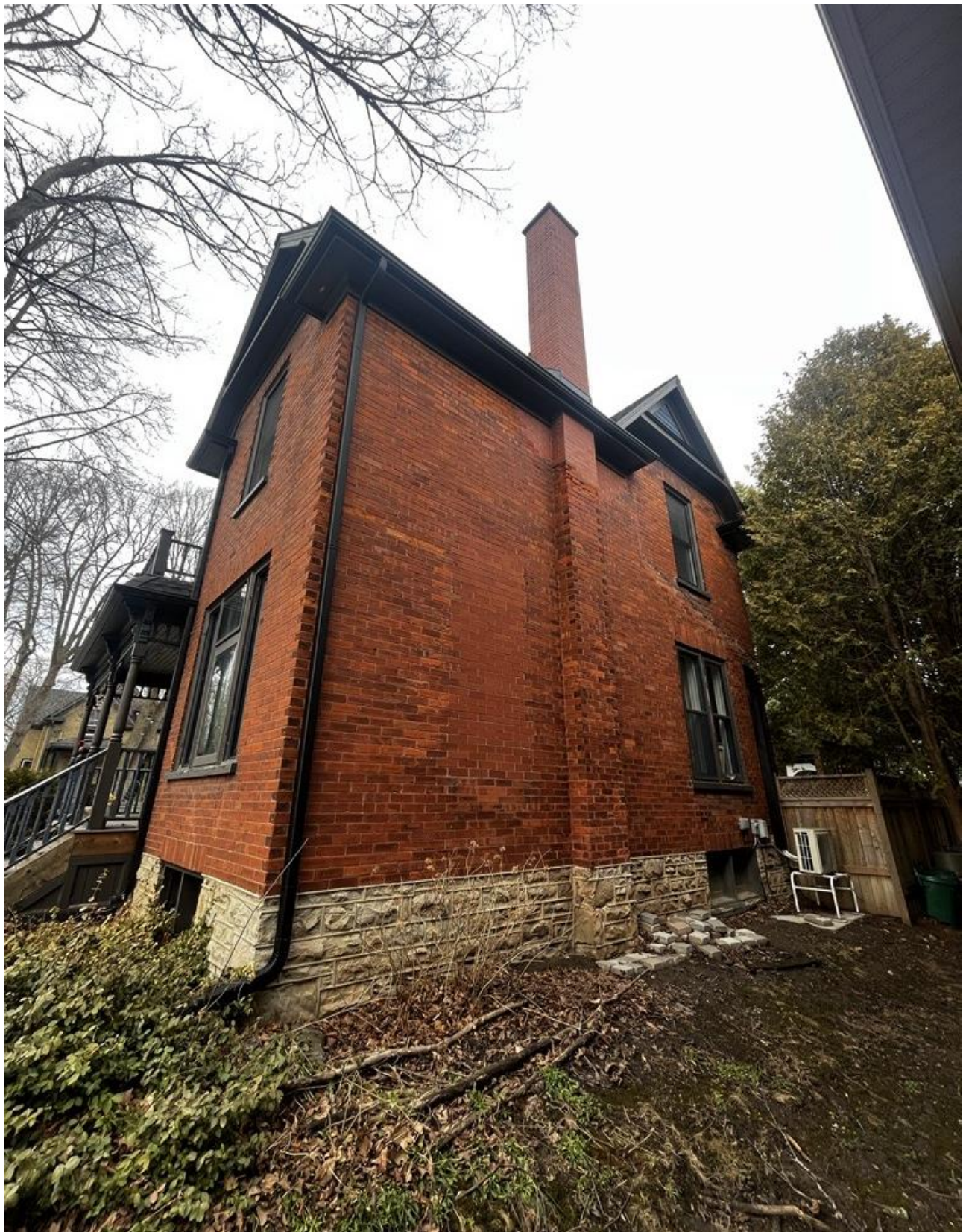
Figure 6: South Side Elevation of Subject Property
