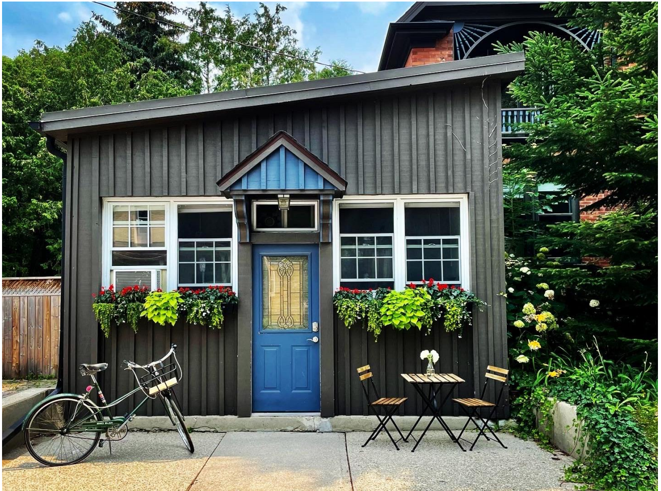
Figure 3: One-Storey Extension Originally Used as the Local Grocers
