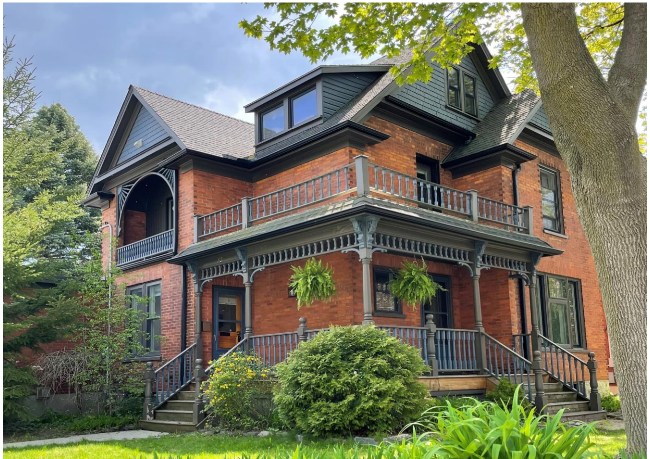
Figure 2: View of the Subject Property
