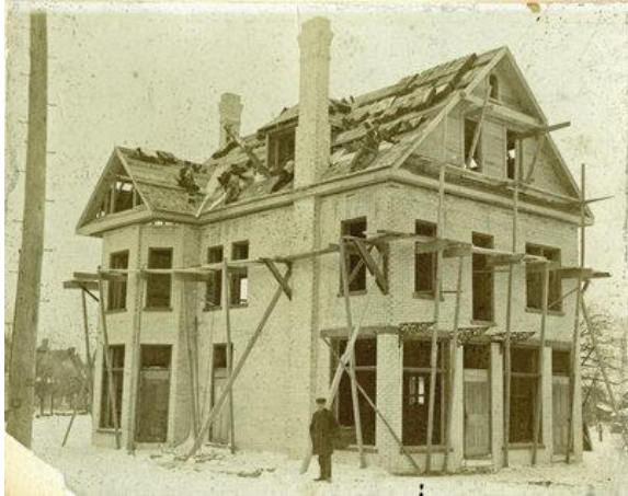
Image 1: Ahrens Five Point Grocery Store, under construction in 1903.
