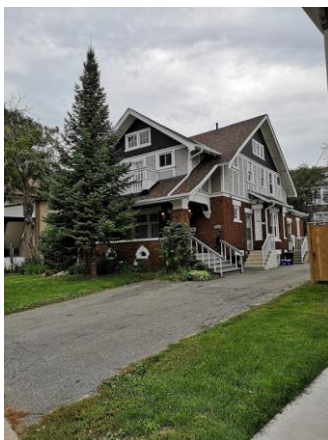
Site Photograph 11: 145 Lancaster Street in similar Craftsman design, slated for demolition.
