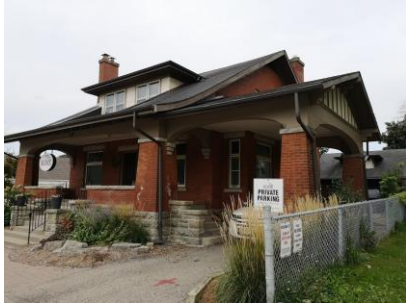
Character-Defining Elements 6: The carport's tapered brick carport columns, flat arch supporting gable.
