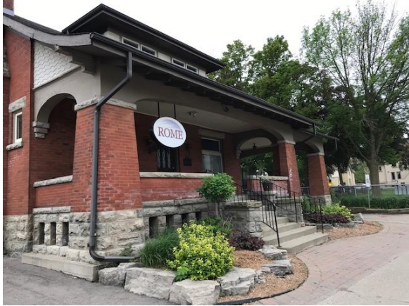
Site Photograph 3: 181 Frederick Street, north elevation.
