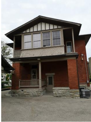
Character-Defining Elements 3: Rear second storey, formerly screened, sleeping porch.
