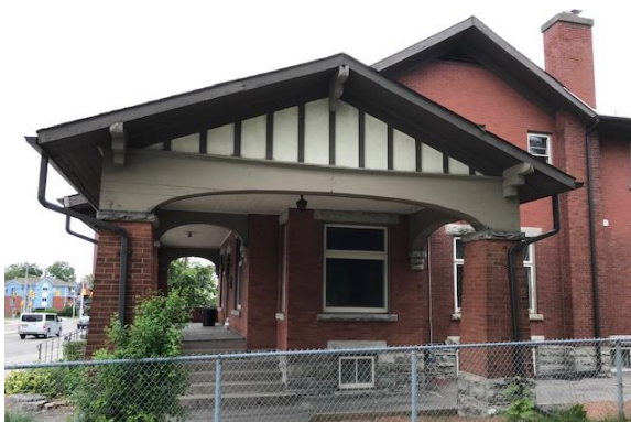
Site Photograph 5: 181 Frederick Street, west elevation.
