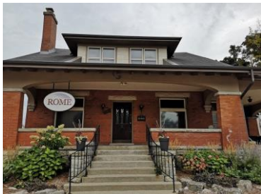
Character-Defining Elements 2: Deep, full-width front porch, supported by tapered brick columns.
