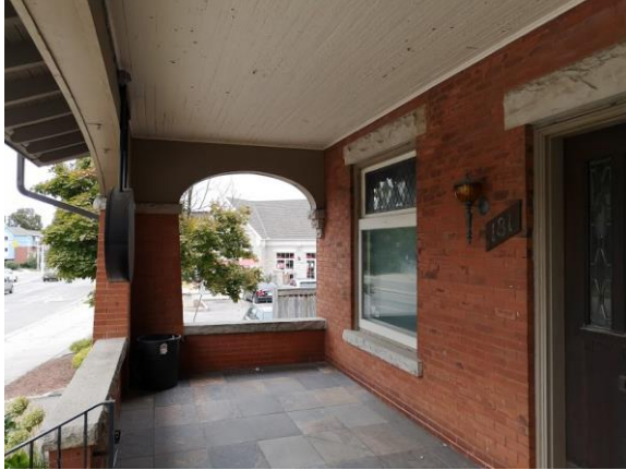
Site Photograph 6: 181 Frederick Street, porch.
