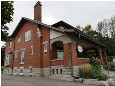
Character-Defining Elements 1: Low sloped main hip roof with bell-cast, deep, bracketed eaves with roof dormer centered on front elevation.
