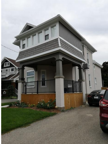
Site Photograph 12: 143 Lancaster Street, slated for demolition.
