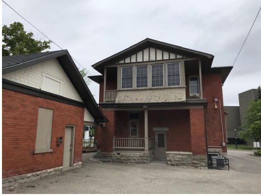
Site Photograph 9: Rear of 181 Frederick Street, South elevation and “Sleeping Porch”.
