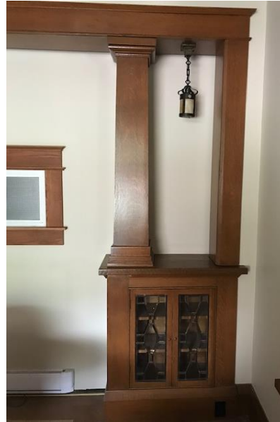
Interior Details 6: One of a pair of square columns and cupboards with glass doors that separated the dining room from the living room. A wall currently fills the former opening.
