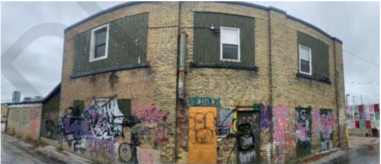
Figure 4: First Addition towards the rear of the property. Source: Draft HIA
