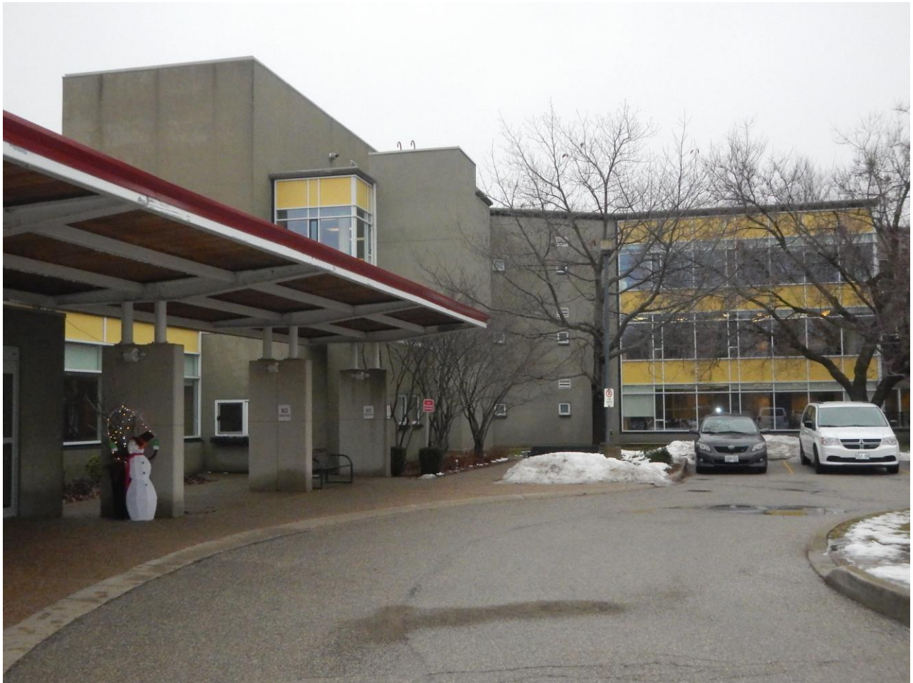
Figure 2: View of the entry canopy with the yellow panels.
