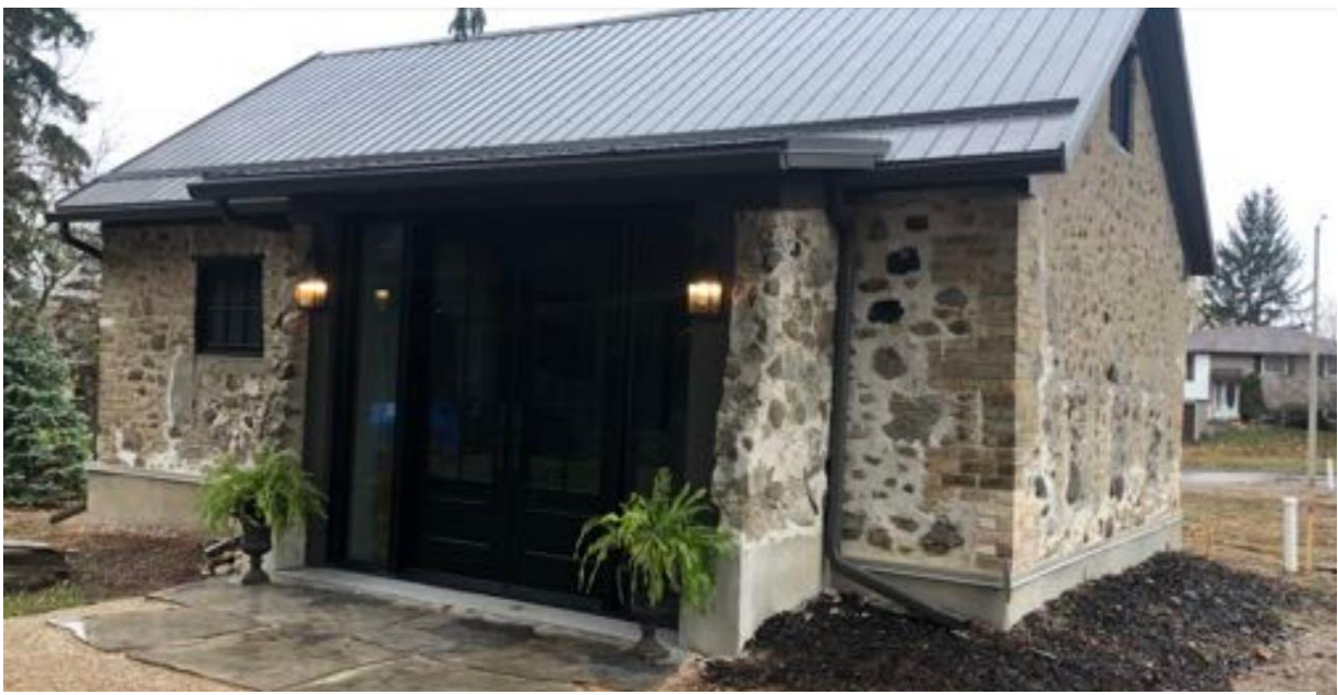
Figure 10: Hog and Hen House After Work
