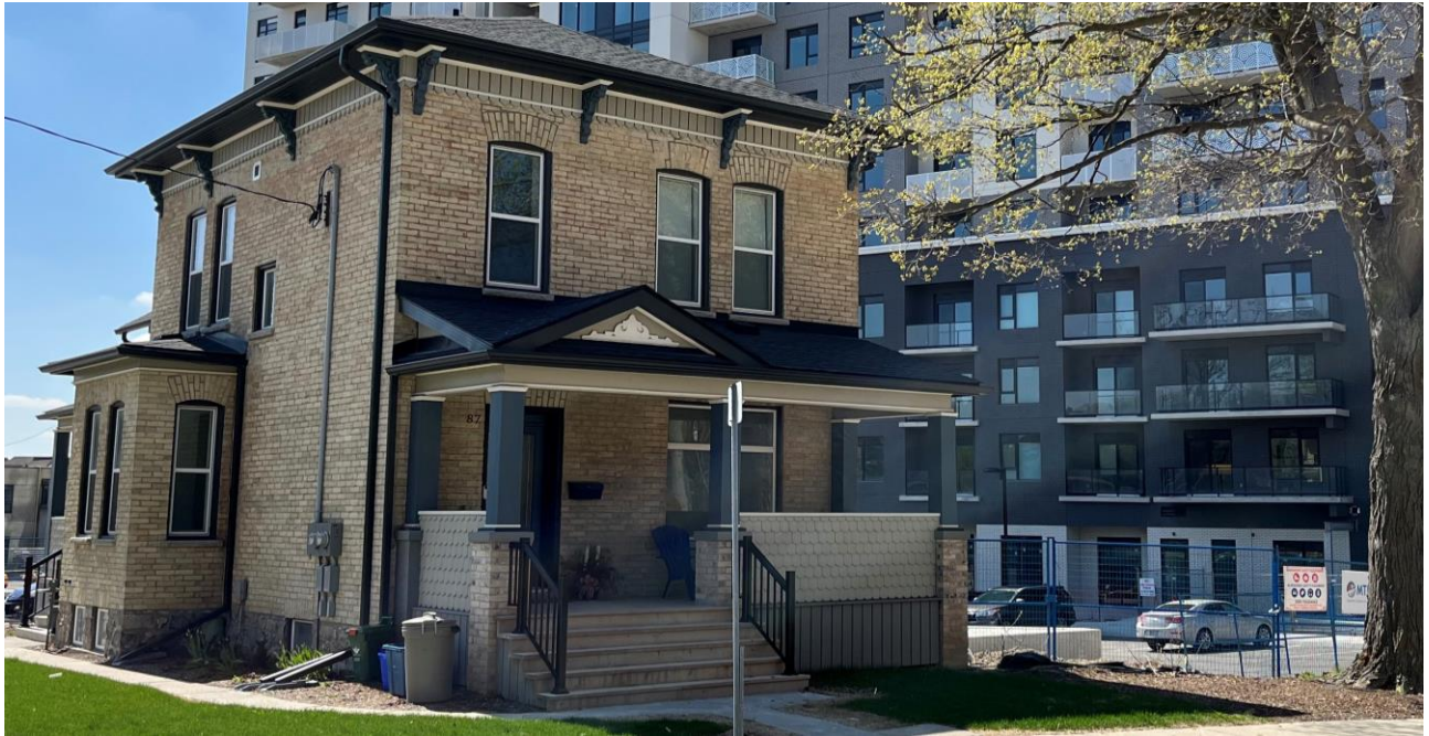
Figure 2: 87 Scott Street After Rehabilitation
