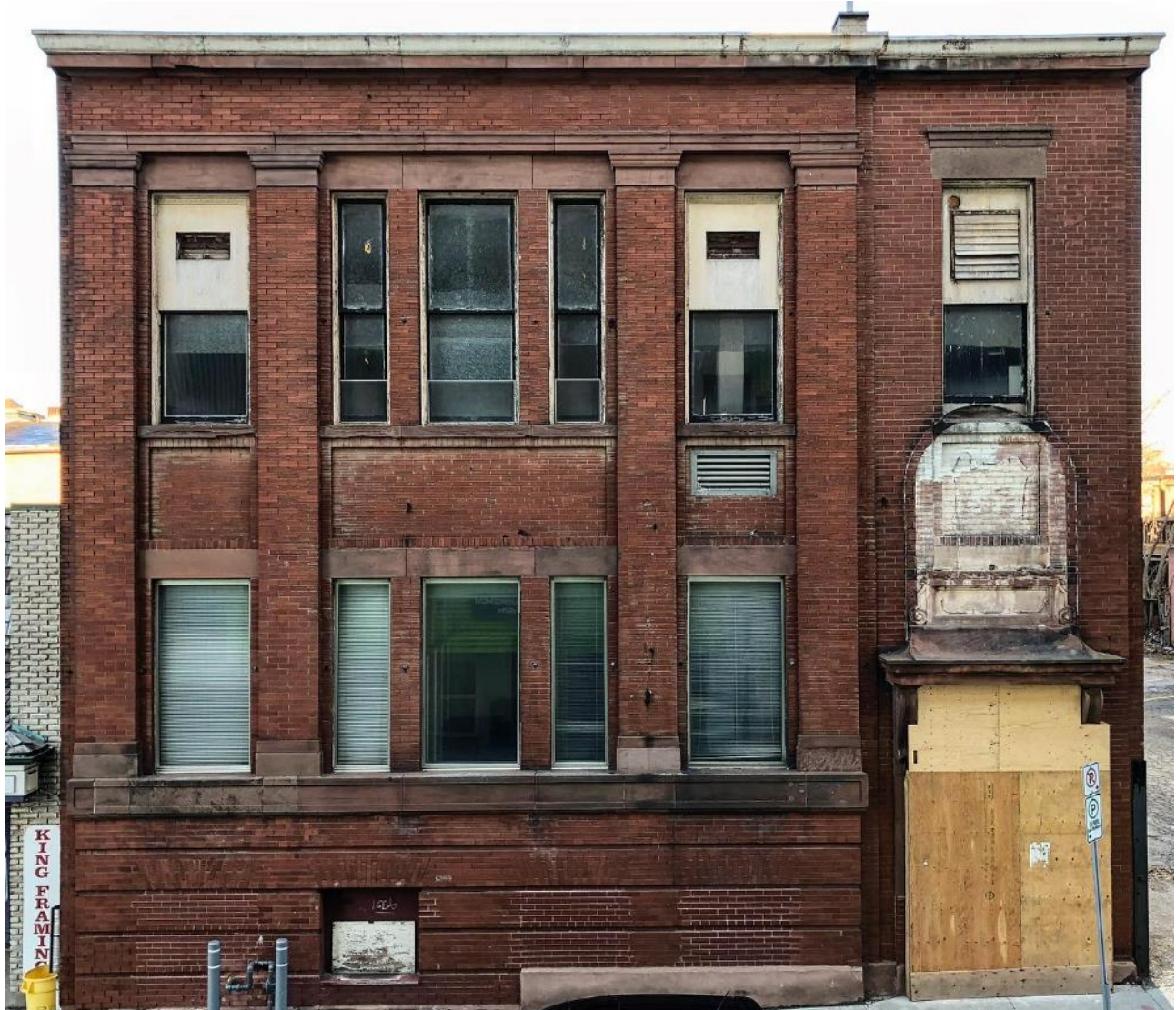
Figure 2: 48 Ontario Street Before Restoration
