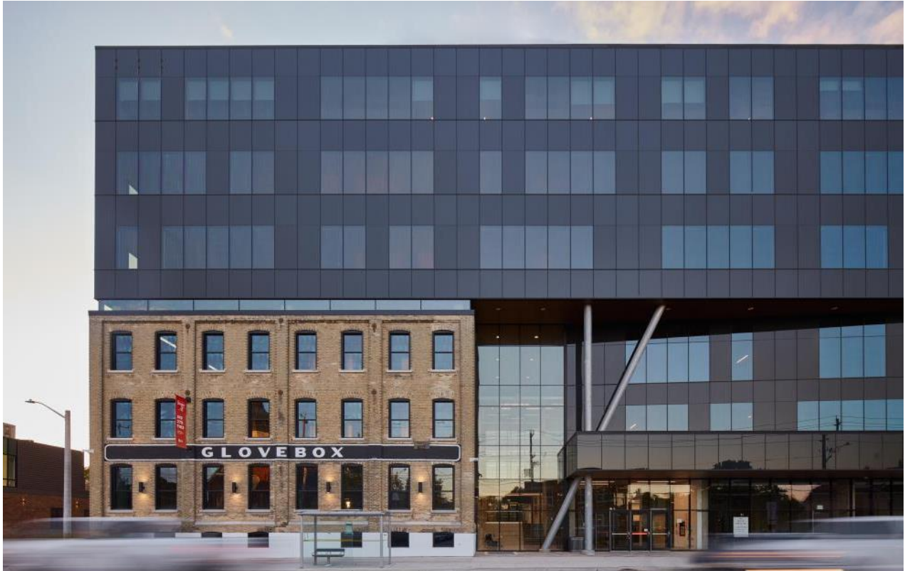
Figure 8: 114 Victoria Street South After Work
