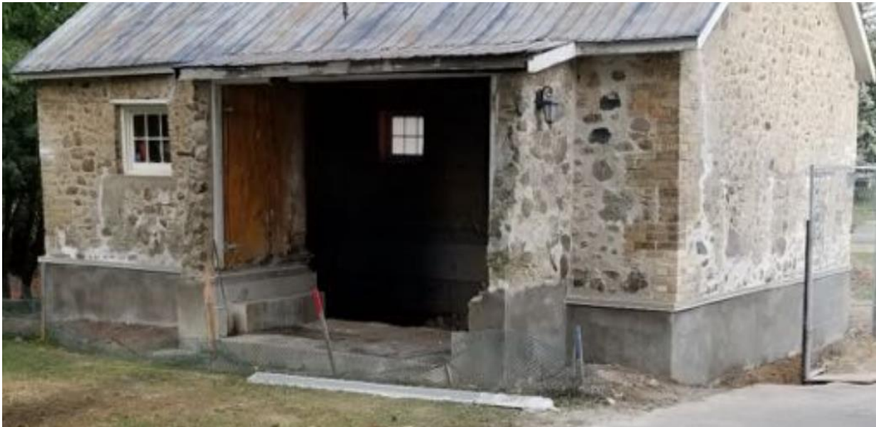
Figure 9: Hog and Hen House Before Work
