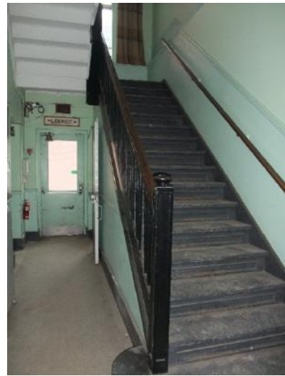
Metal balustrade and newel-post, slate treads and metal risers
