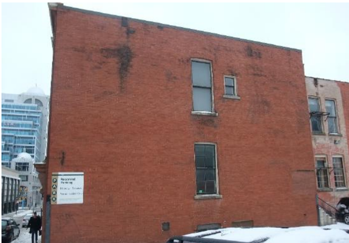
Partial North façade; location of two new windows.
