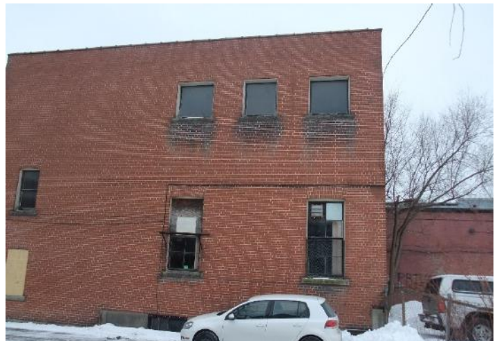
Partial North façade; location of one new window.
