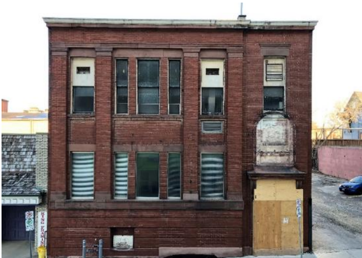
East Elevation, Ontario Street, showing existing door and windows.
