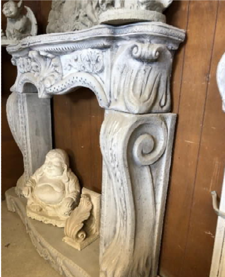
Example of level of detail to be achieved with replacement pre-cast concrete. Existing entablature and frontispiece to be used in creating formwork.
