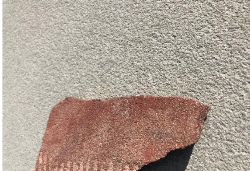
Texture of new pre-cast concrete (beyond) compared to existing frontispiece (front).
