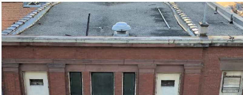
Brownstone fascia band along roofline.
