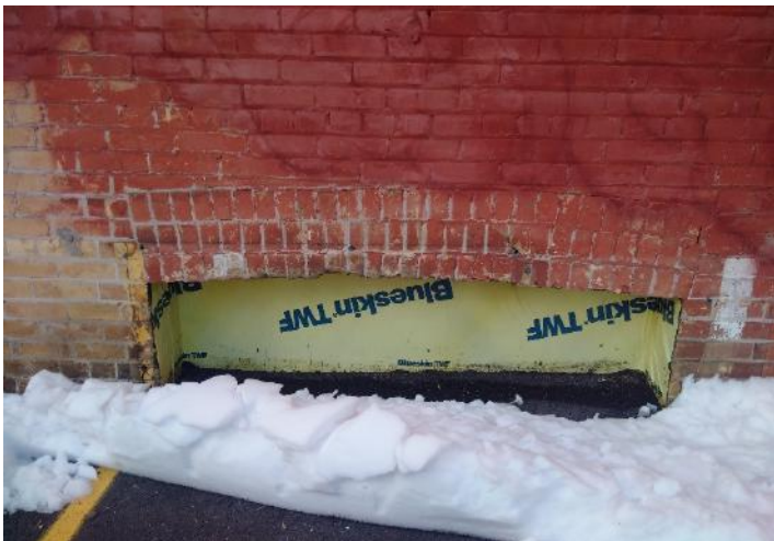
Wide, low window (hidden by black car on Partial North Elevation on previous page). Existing opening to be infilled with recessed brick.
