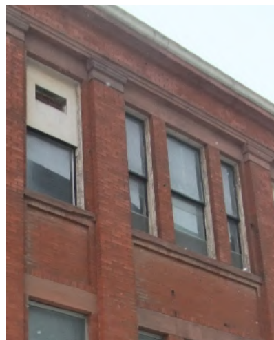
Detail photo of East Elevation, existing brownstone sills.
