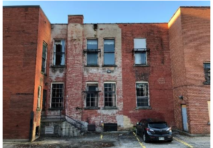
Partial North Elevation, showing existing doors and windows.
