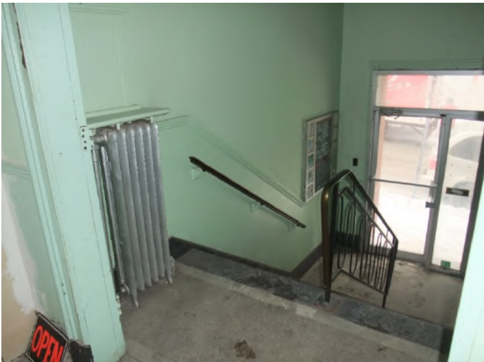
Main entrance stair and terrazzo floor
