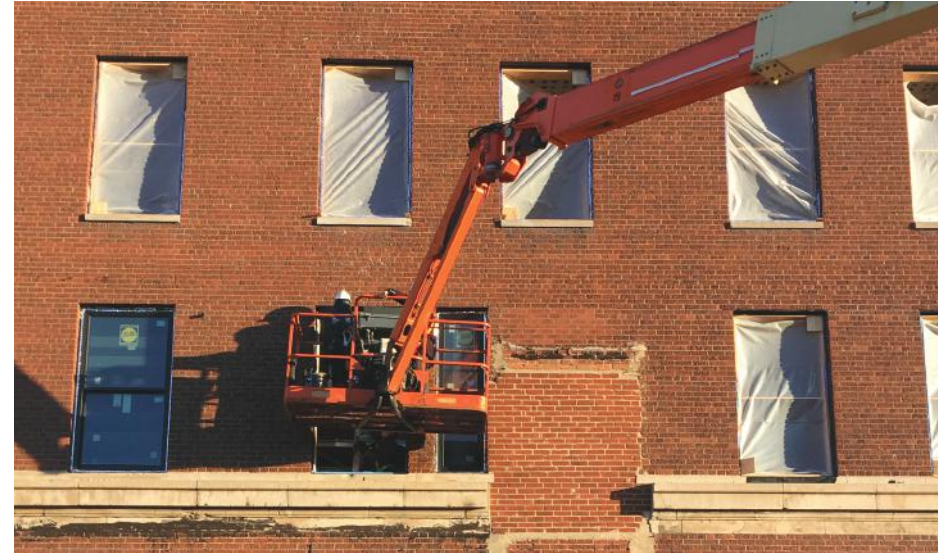
Photo: Installation of Double Hung Windows at the Westinghouse, Hamilton
