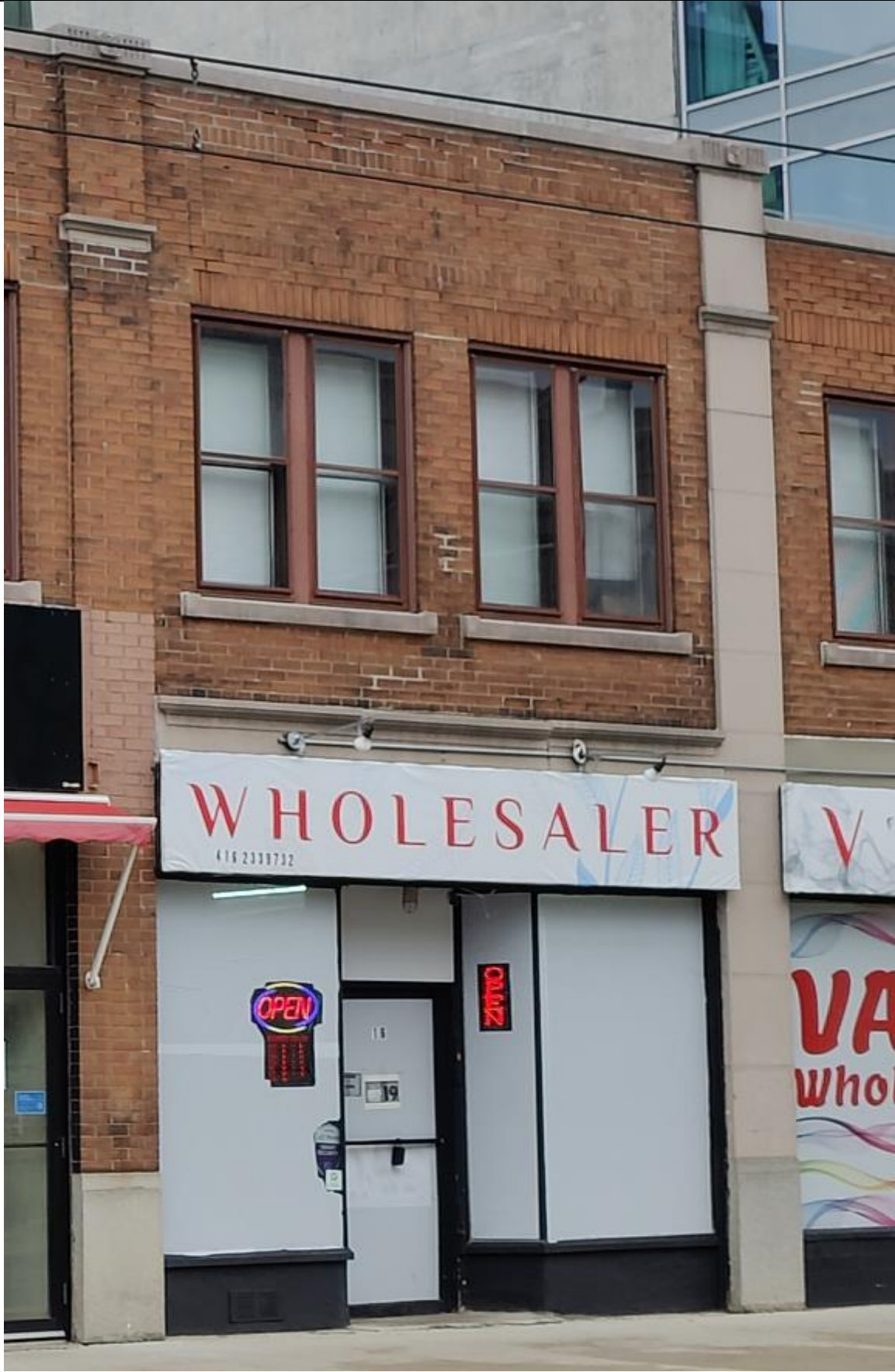
Close up of one bay displaying the different pilasters and decorative brickwork above the second-storey windows
