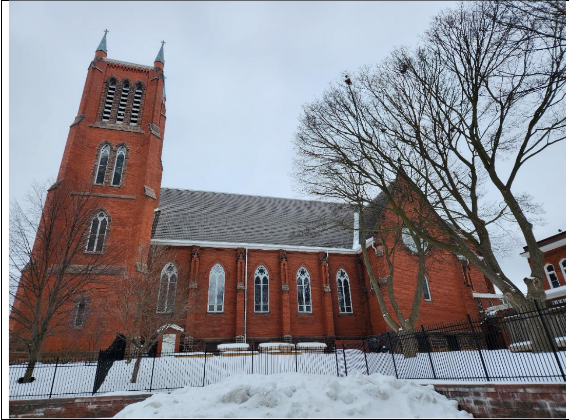
73 Young Street – South Façade (looking towards Duke Street)
