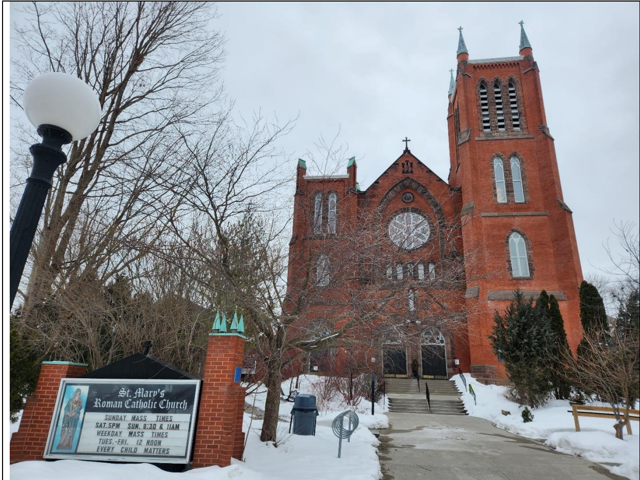
73 Young Street – Front (west) Façade
