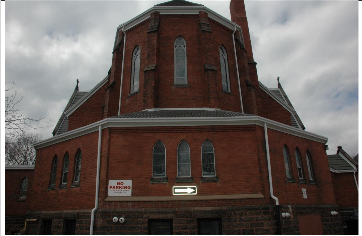
73 Young Street –East Façade (looking towards Ontario Street North)
