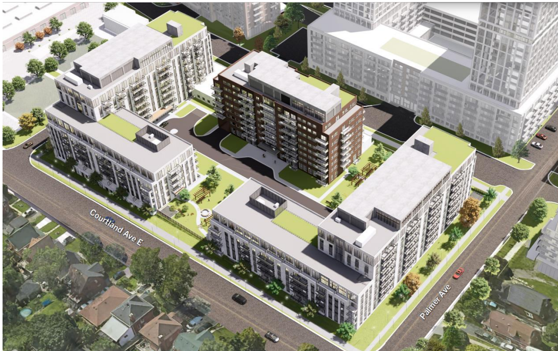
Figure 17: Aerial Rendering showing the mid rise building step backs from 5 storeys to 8 storeys along Courtland Avenue East.
