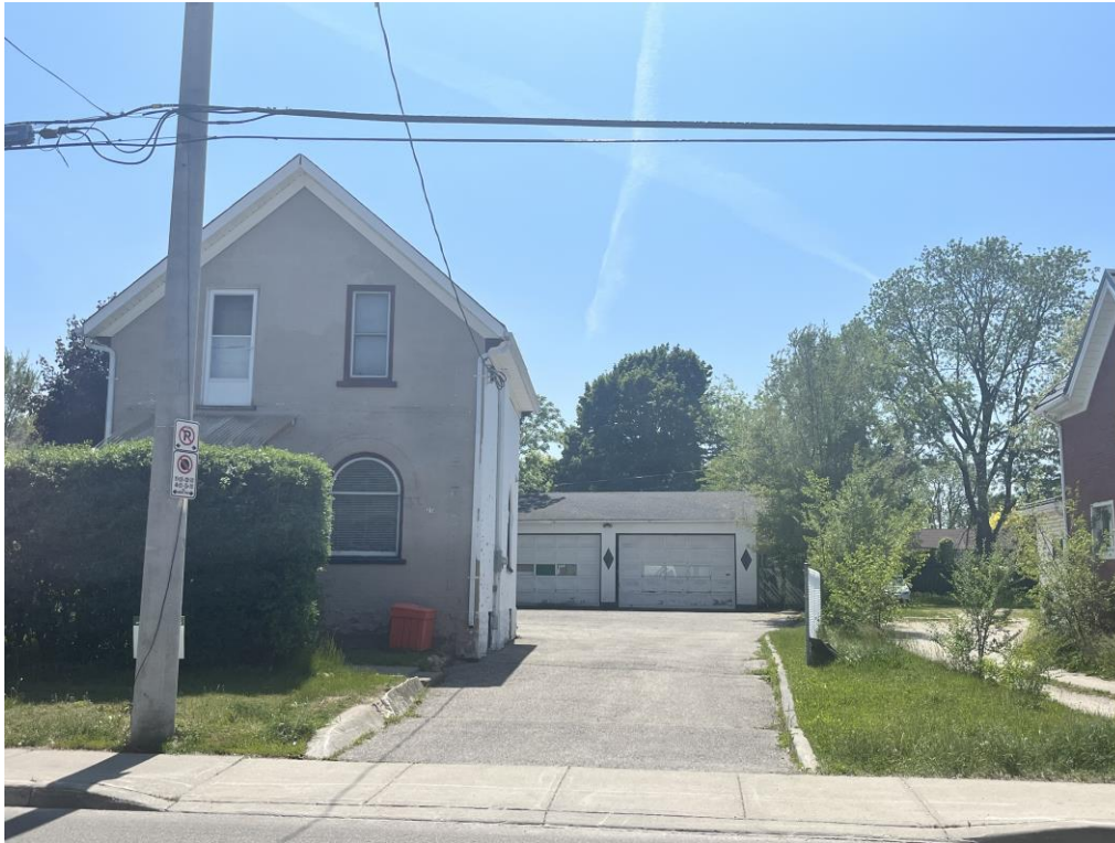
Figure 4 – Front View Photo from Site Visit
