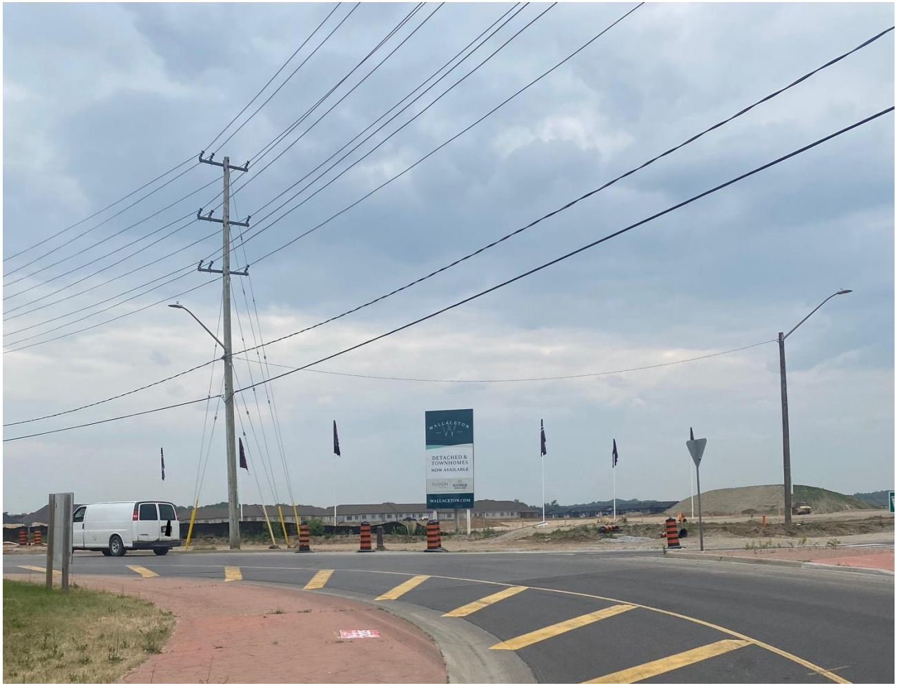
Figure 2: Existing site conditions at 1950 Fischer Hallman Road
