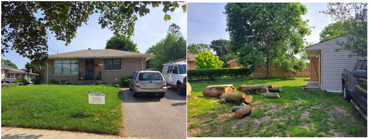
Figures 2 and 3: Front of Subject Site (Left) and Location of Future Detached Garage (Right)
