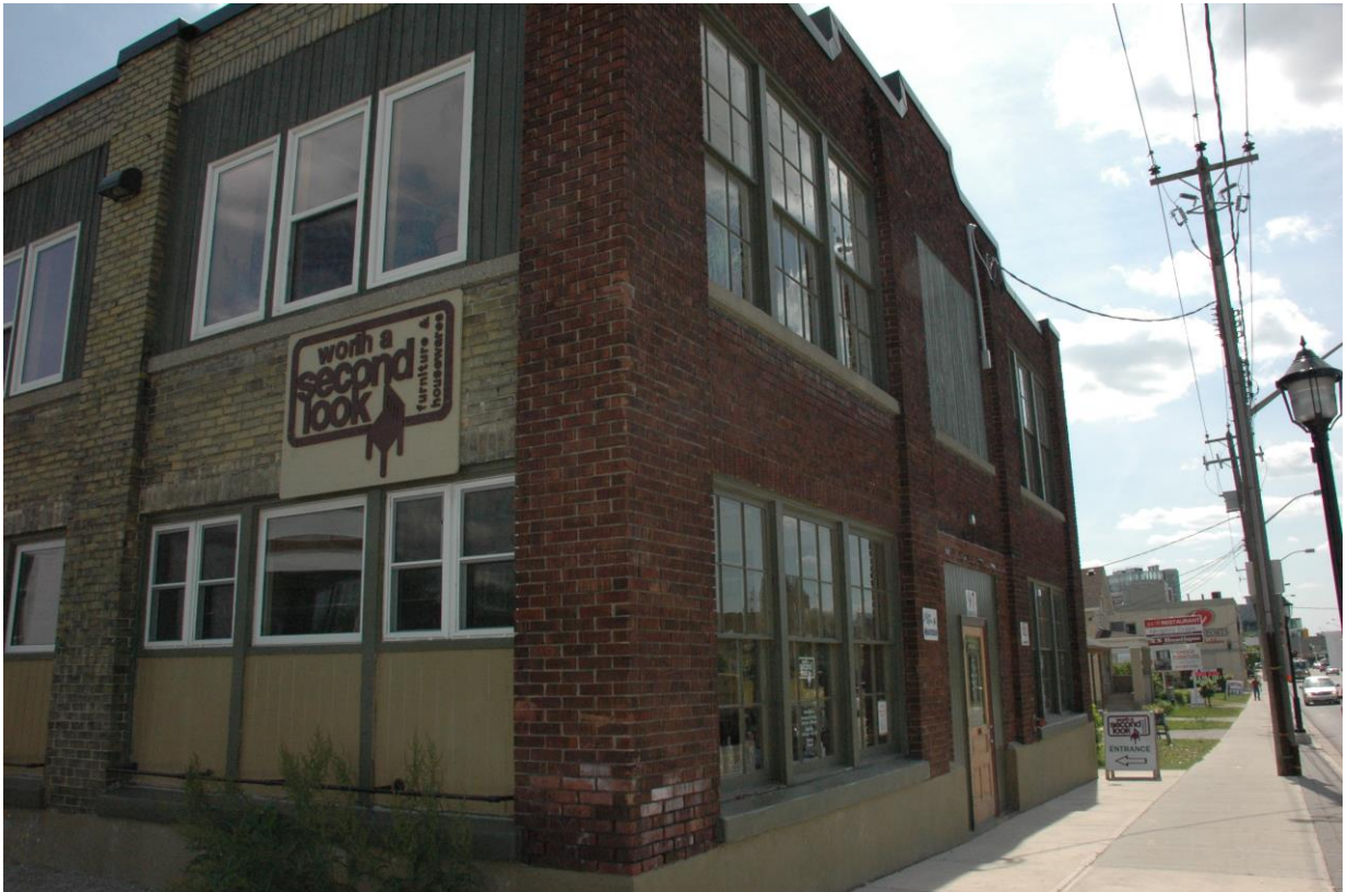
Figure 3: Front and East façade of 97 Victoria Street North.
