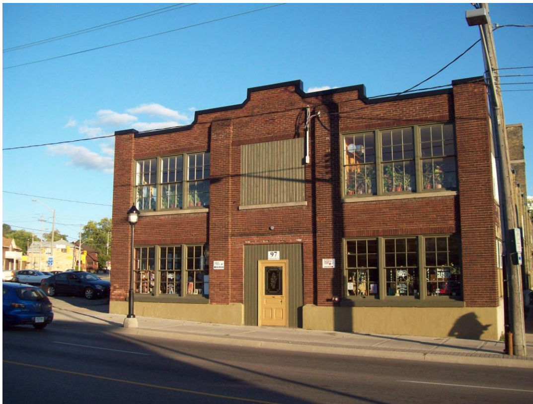
Figure 2: Front façade of 97 Victoria Street North.
