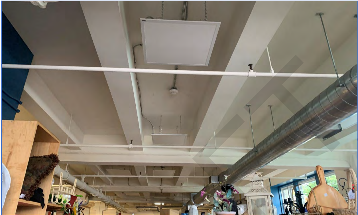
Photo 11: View southeast showing the building's structural, mechanical, electrical, and plumbing systems
