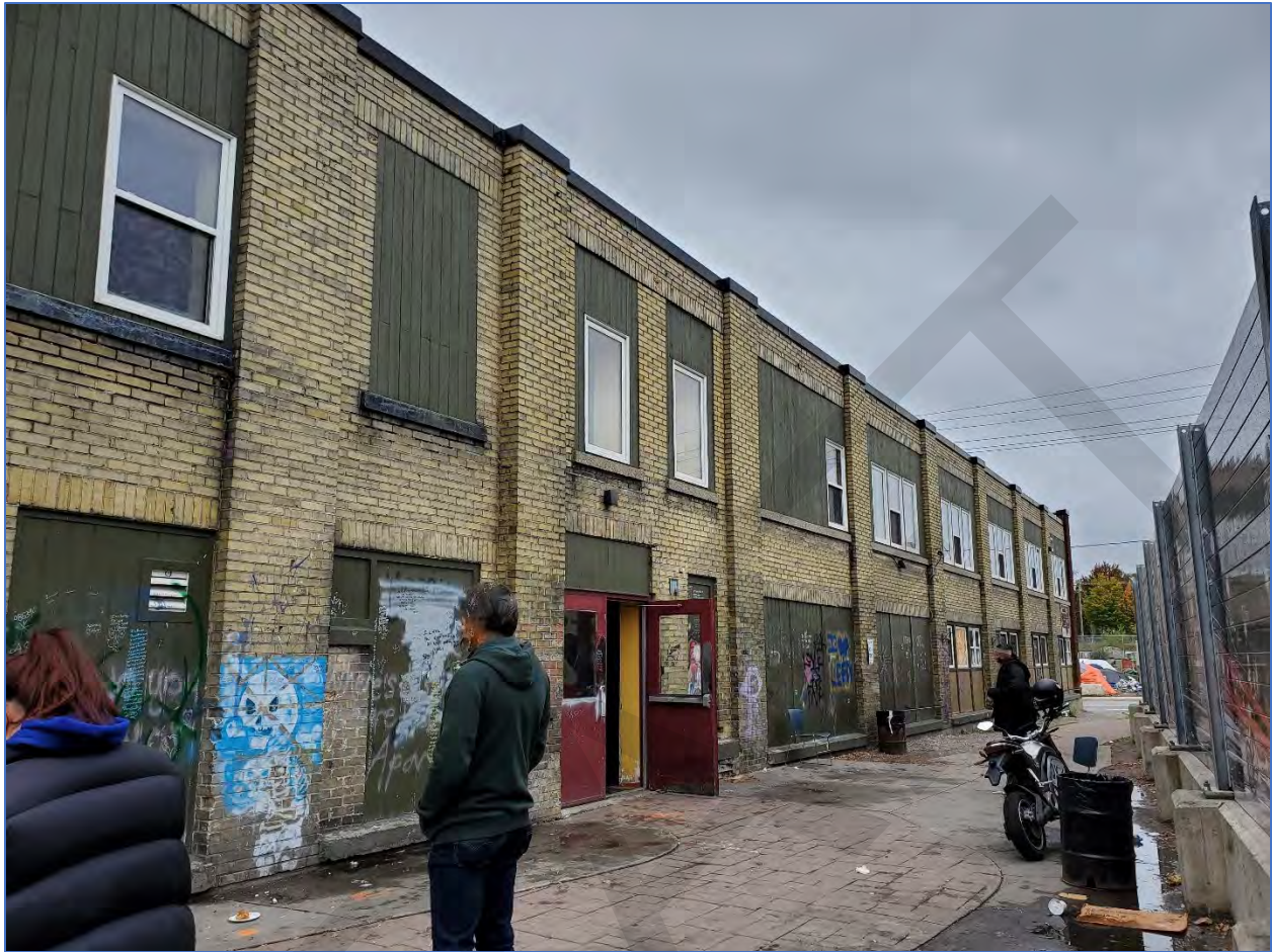
Photo 5: View west showing the Property's northeast elevation
