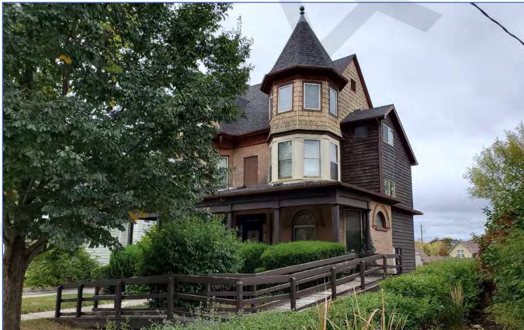
Photo 21: View northwest showing 70 Francis Street North's southeast and northeast elevations
