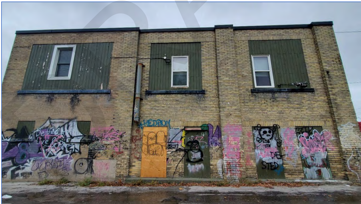
Photo 8: View northwest of the Property's southeast elevation. The addition on the right follows the same rhythm of bays and buttresses found along the other elevations. The addition to the left is void of buttresses and is a distinctly different colour
