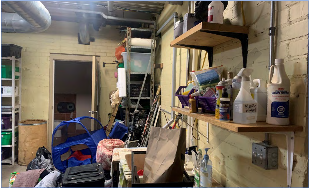
Photo 15: View showing painted brick walls
