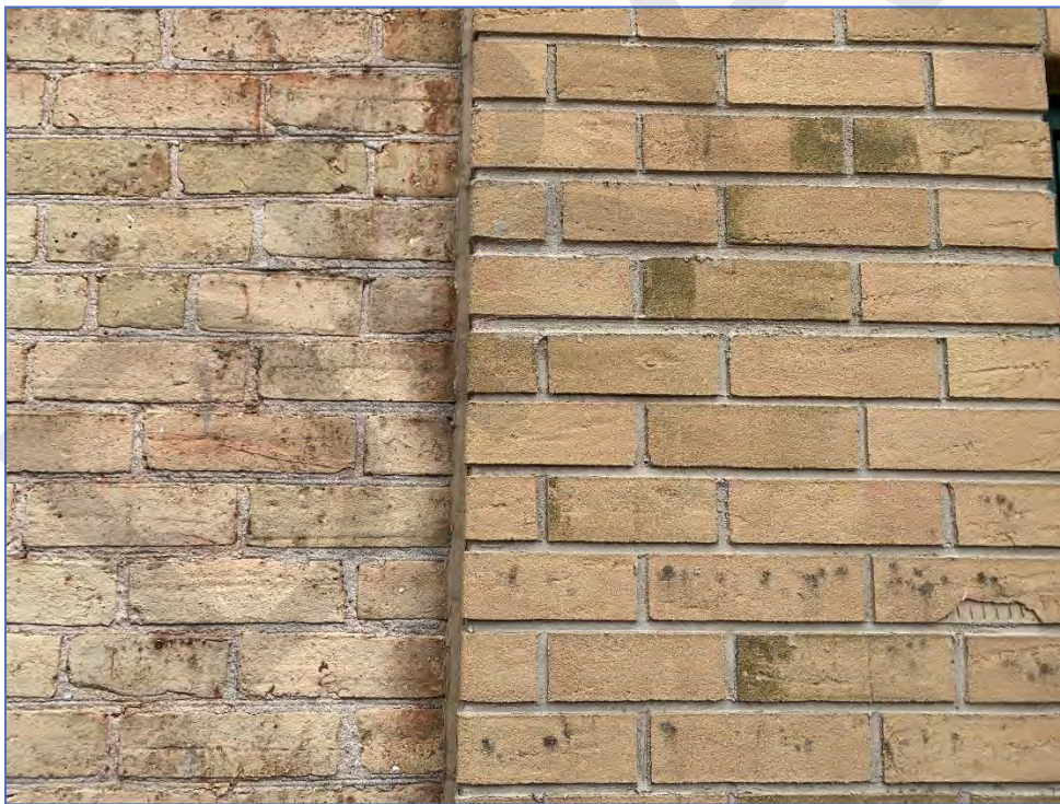
Photo 3: Detail of materials, original yellow brick (left) and faux yellow brick finish (left). The result is an addition that is compatible with the earlier structure, and distinguishable as a modern addition
