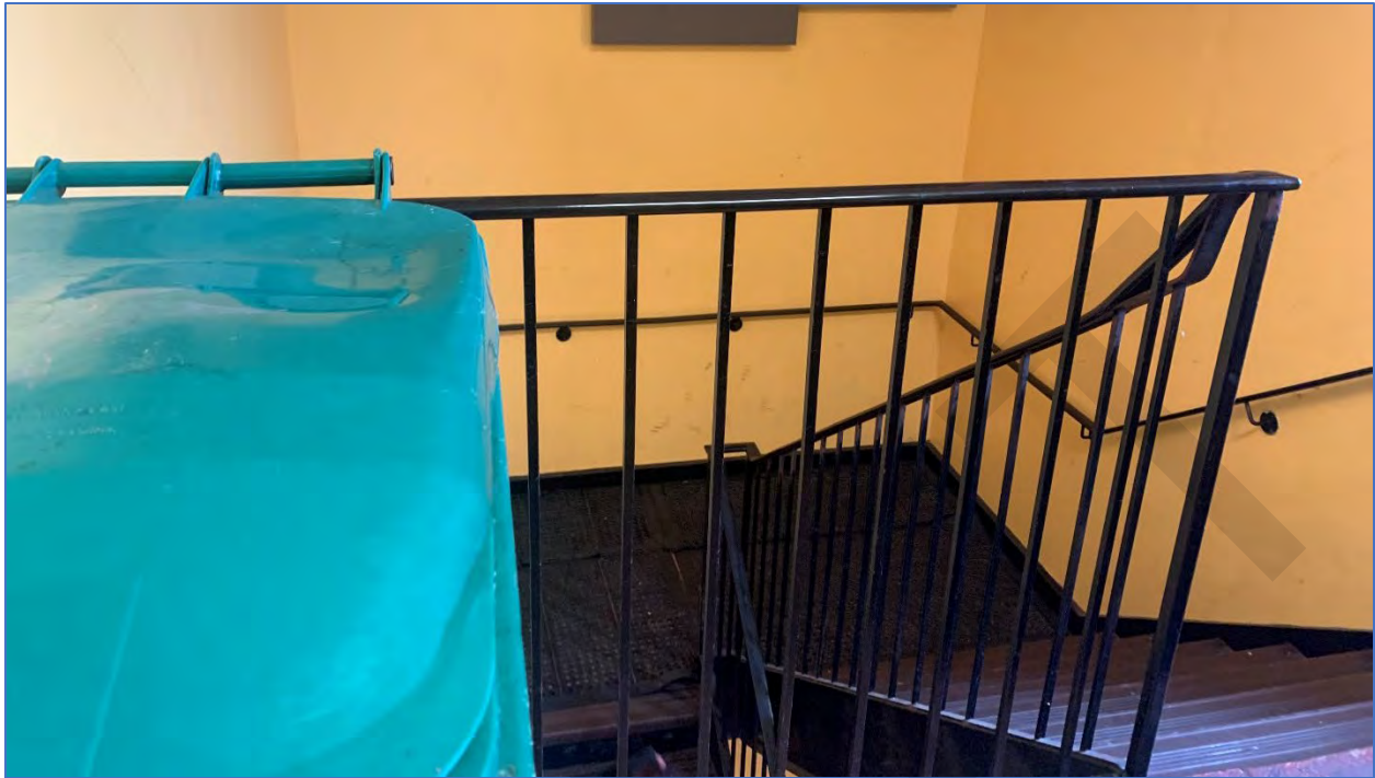
Photo 17: View northwest showing the staircase providing second floor access
