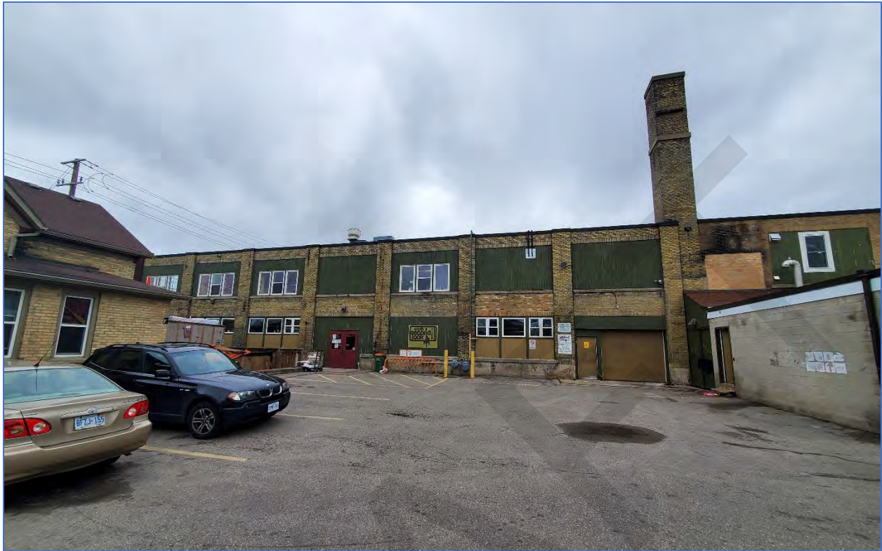
Photo 7: View northeast showing the Property's southwest elevation
