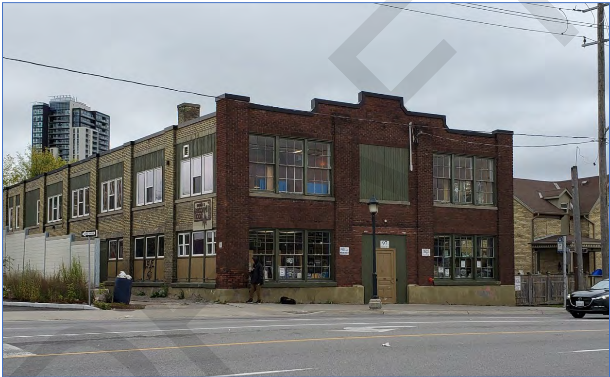
Photo 4: View south showing the Property's northwest (primary) and northeast elevations
