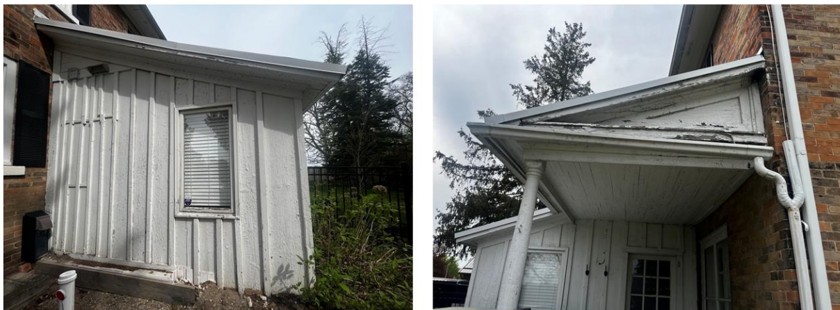
Figure 3: Existing Rear Addition to be Demolished
