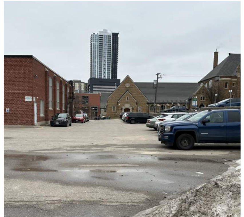
Figure 7. View of the asphalt parking lot at the rear of the site looking north towards Church Street entry/exit to the site.
