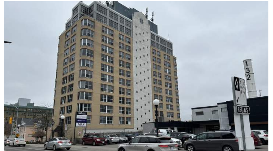
Figure 11. View of the adjacent apartment building along Queen Street looking west from the subject site.
