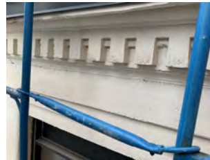
CONCRETE CORNICE DETAIL
