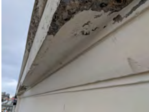
CONCRETE CORNICE DETAIL
