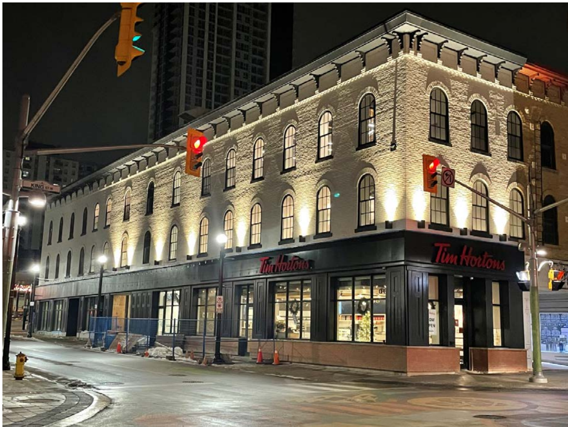
Figure 2: 1 Queen Street North After Restoration
