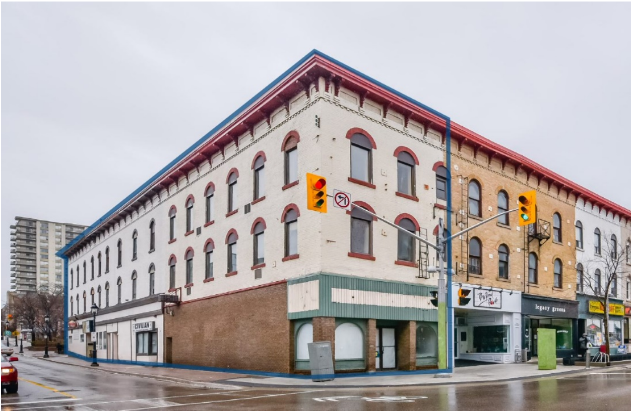
Figure 1: 1 Queen Street North Before Restoration
