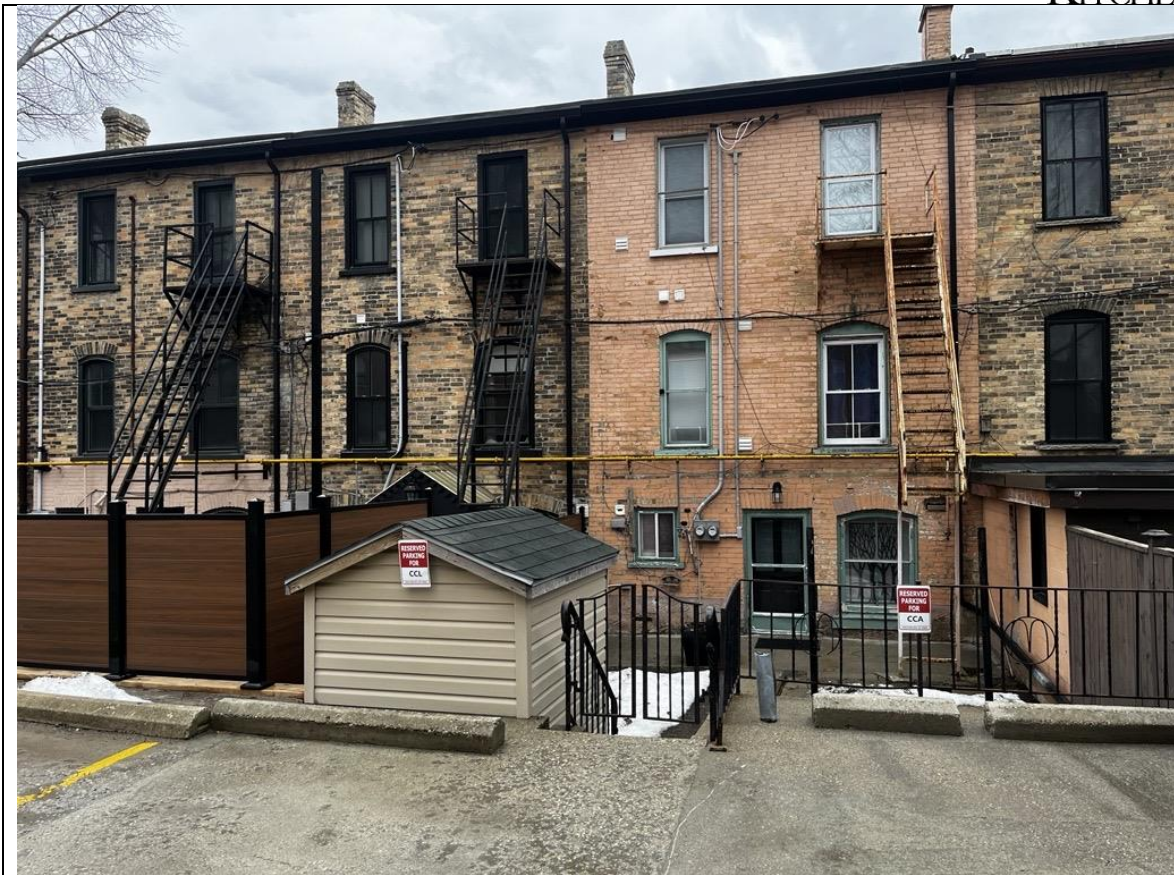
Rear Façade of 26 Courtland Avenue East
