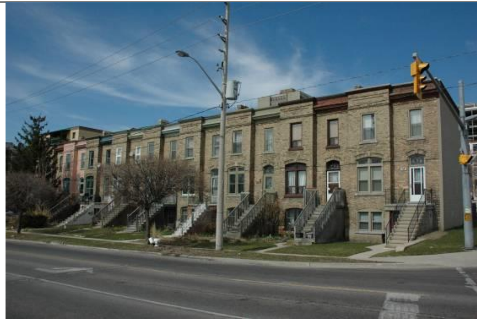
26 Courtland Avenue East – Entire Nelson Terrace Row House Building
