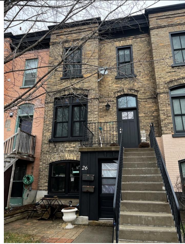
Front Façade of 26 Courtland Avenue East
