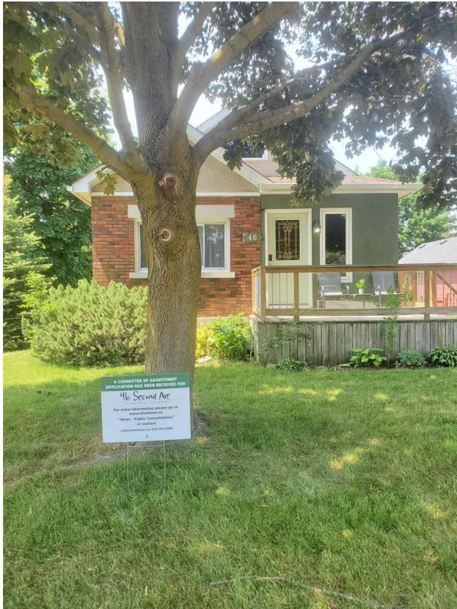
Figure 2: View of Existing Detached Dwelling
