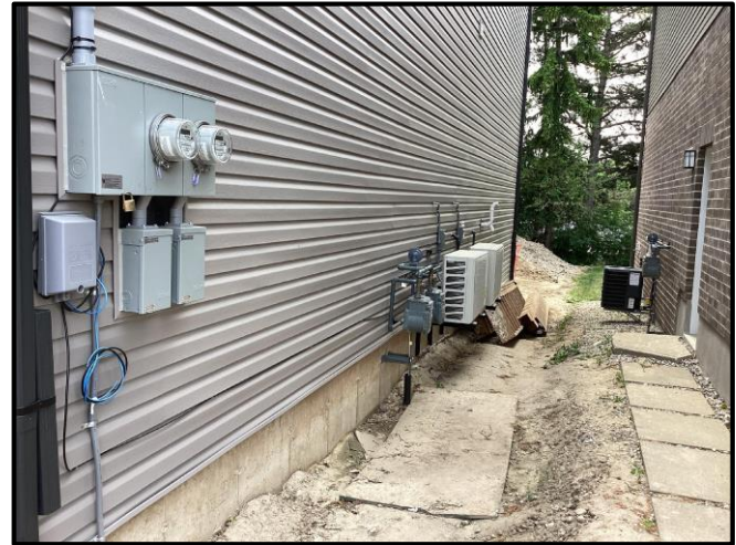
Figure 4: The east side yard
