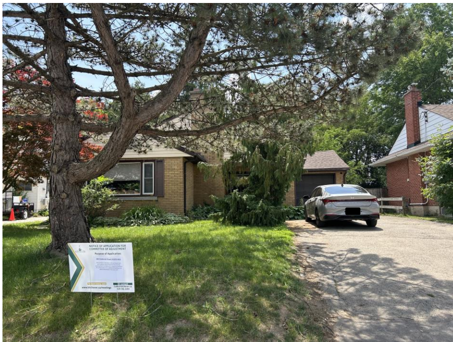
Figure 2: Front view of the property during site visit
