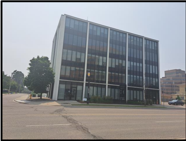
Figure 3 - The front view of the building, which will contain the proposed restaurant patio
