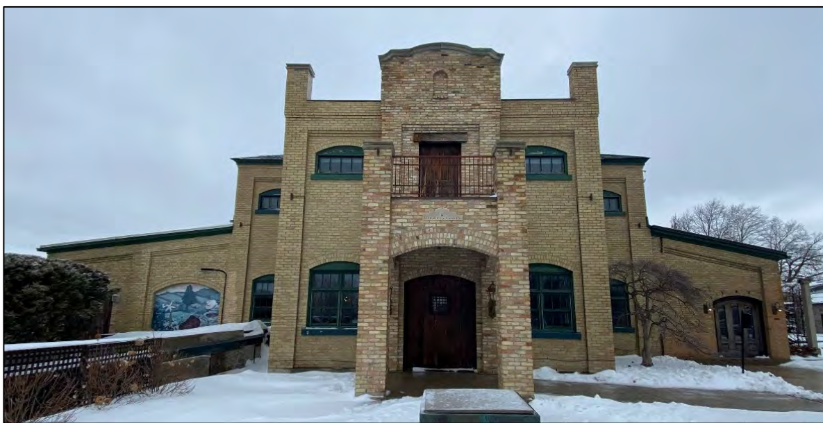
Figure 23: South elevation of warehouse building (Building 1) (MHBC, 2023).
