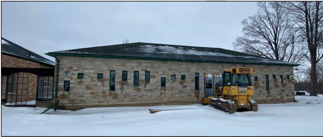
Figure 40: Image of west elevation of Building 3 (MHBC, 2023).
