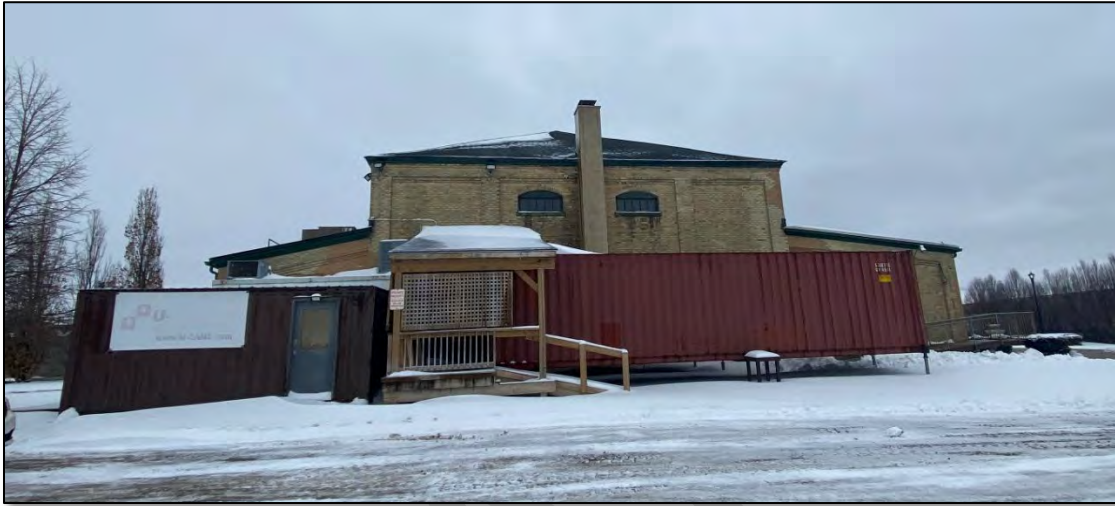
Figure 28: Image of north elevation of main building (MHBC, 2023).
