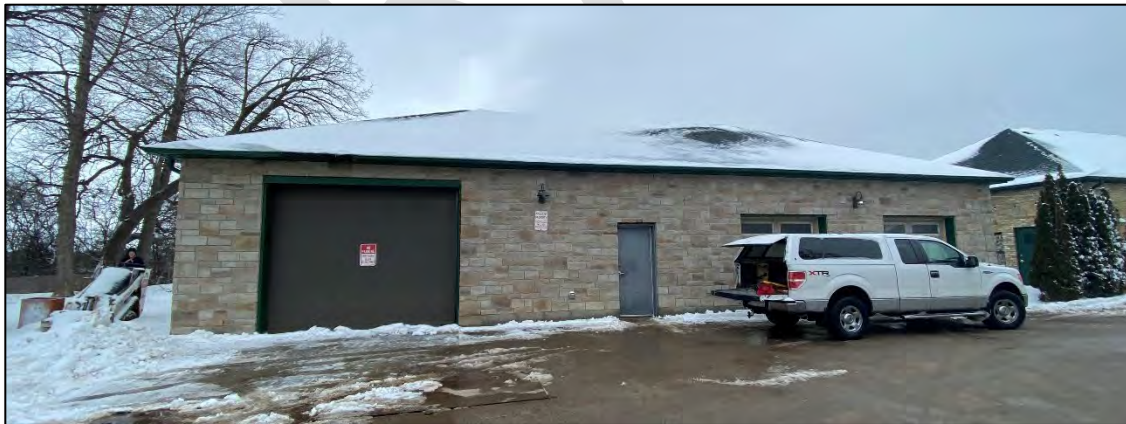
Figure 37: Image of west elevation of Building 3 (MHBC, 2023).
