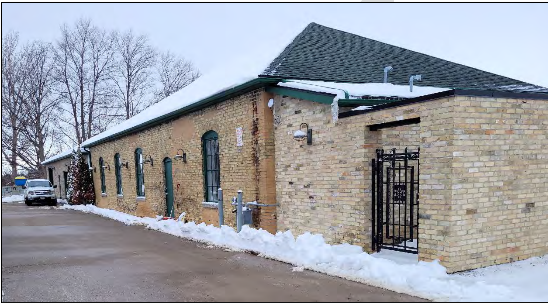
Figure 33: Image of southwest corner of Building 2, showing west elevation (left) and south addition (right) (MHBC, 2023).
