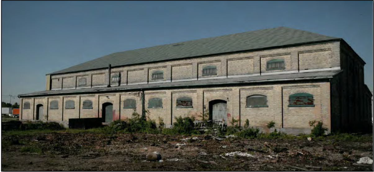
Figure 15: Image of building prior to 2005 alterations, facing southwest (provided by owner).
