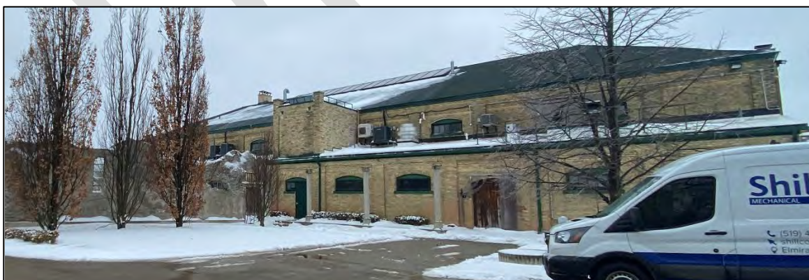
Figure 27: Image of east elevation of Building 1 (MHBC, 2023).
