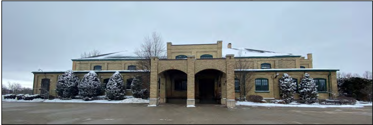
Figure 30: Image of west elevation of main building (MHBC, 2023).
