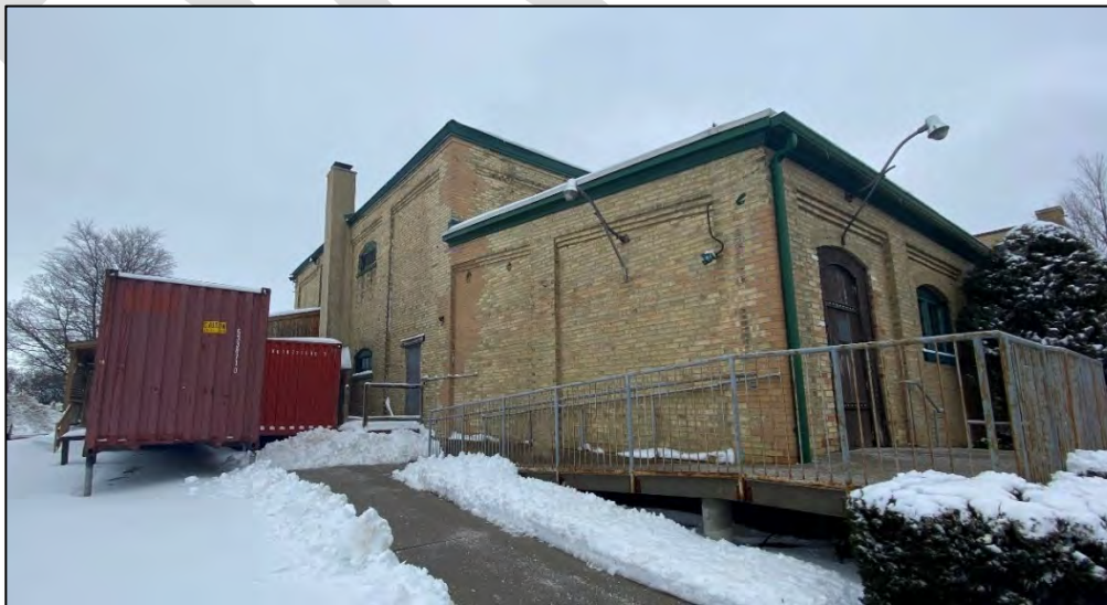
Figure 29: Image of northwest corner of building and external storage structures (MHBC, 2023).
