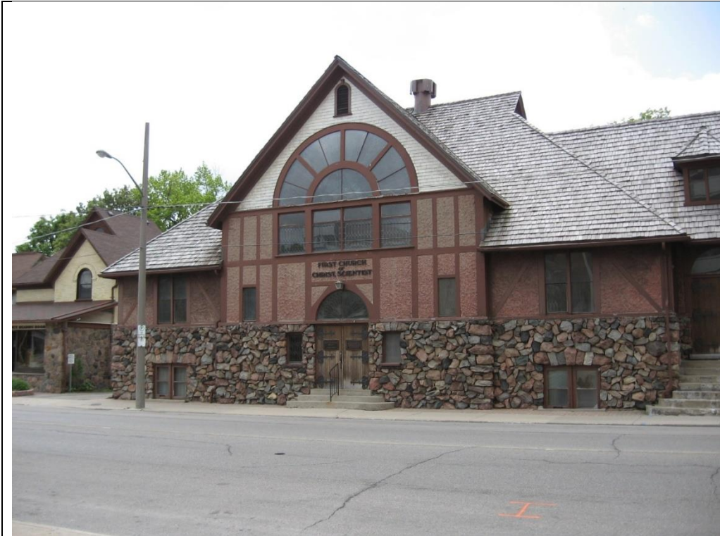
Water Street North Elevation
