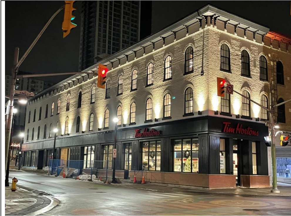
4-30 King Street East/ 1 Queen Street North – Front Façade
