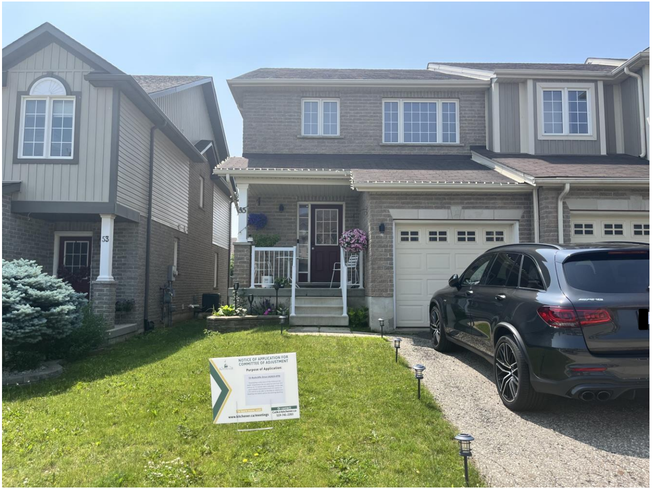
Figure 4 – Front View Photo from Site Visit
