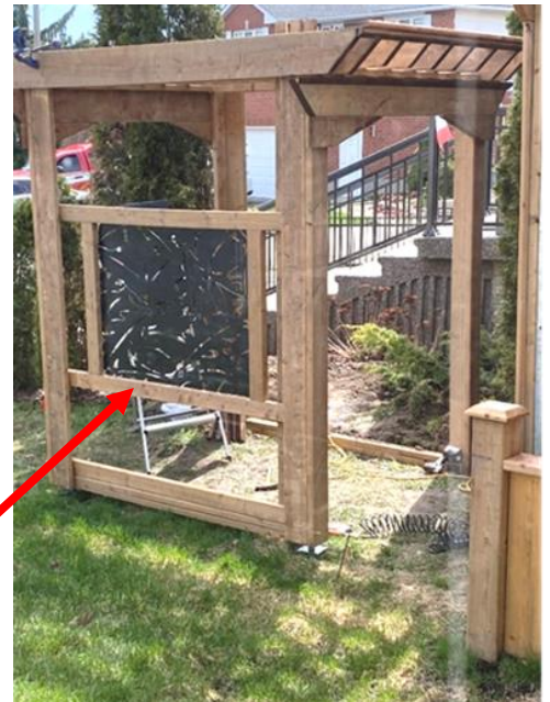
Above: ornamental metal insert. Once the north-side was covered with lumber, the insert became visible only for the Applicants.
