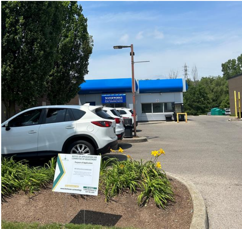
Figure 2: Front view of building during site visit
