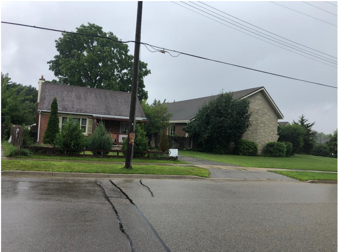
Figure 5: View of Existing Lot 110-116 Hoffman Street (July 27, 2023)
