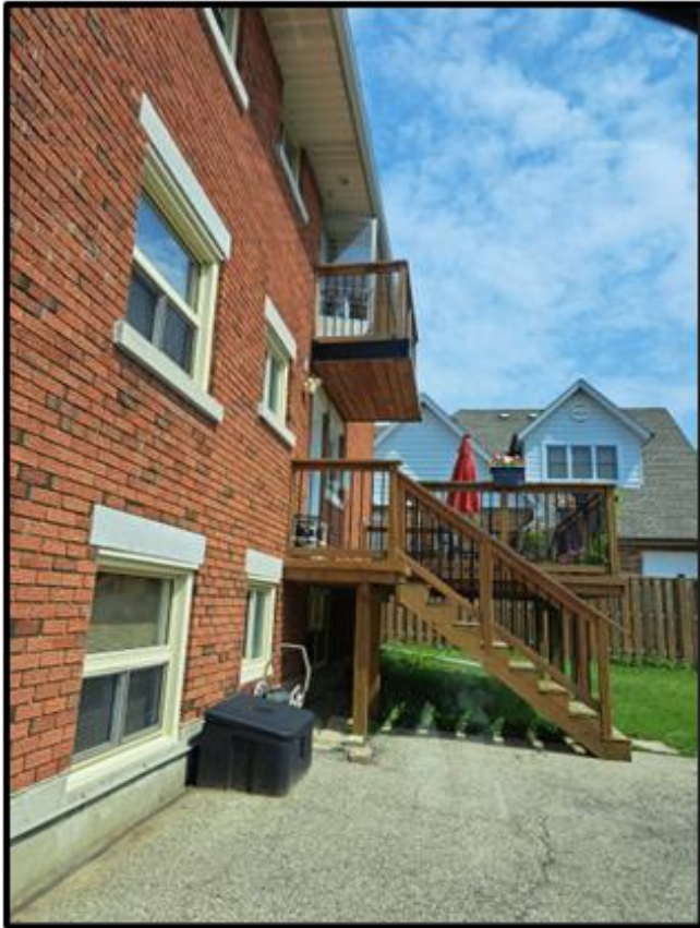
Figure 5: The existing rear elevation where the proposed addition will be attached
