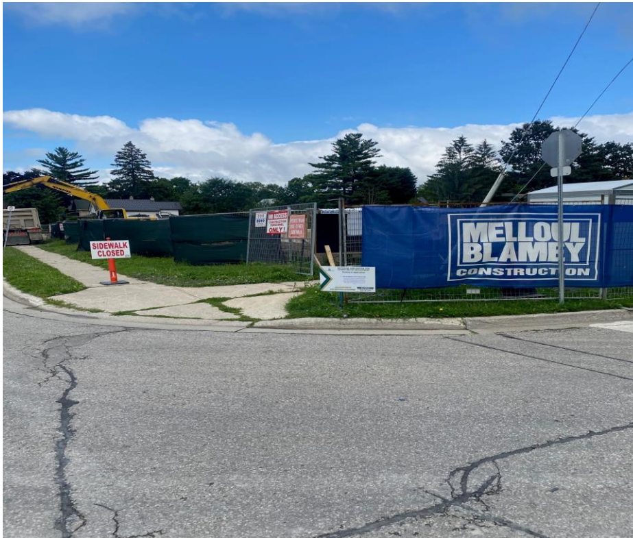
Figure 2: Existing site conditions at 134-152 Shanley Street
