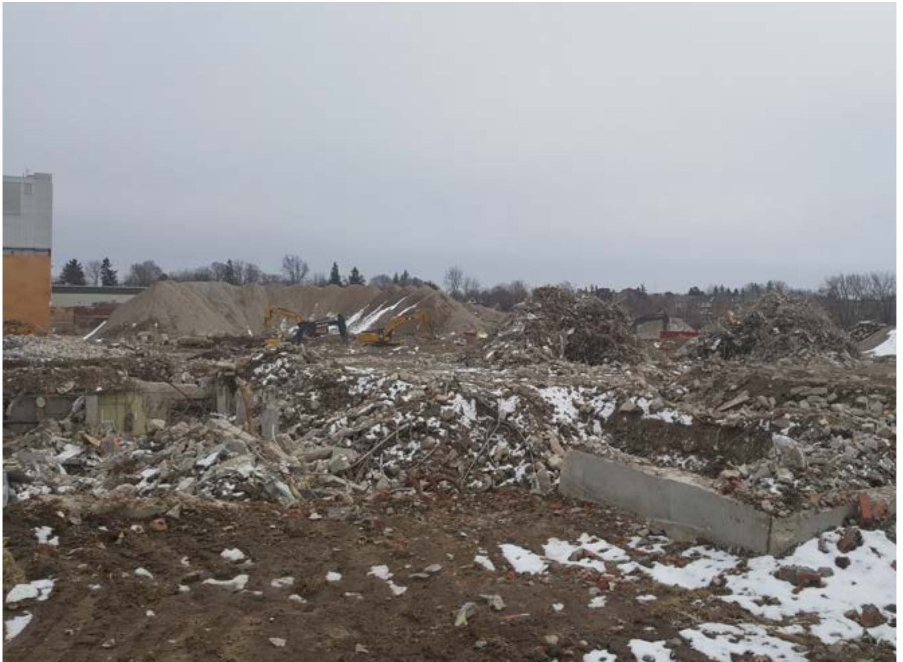
Site Demolition Underway
