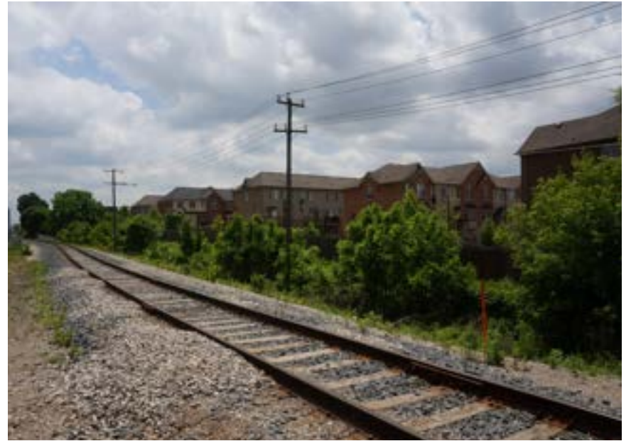
CN Rail Corridor and Townhouse Block abutting the south side of the Site
