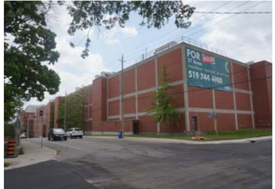
Former Plant Building on Courtland Avenue East
