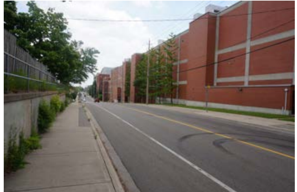
Courtland Avenue East Streetscape (pre-demolition)
