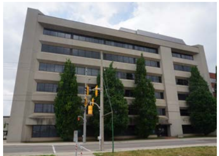
Existing Office on Courtland Avenue East
