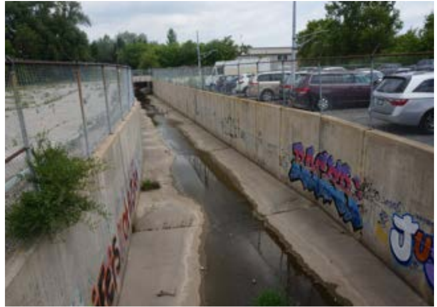
Schneider Creek Culvert north of Courtland Ave E
