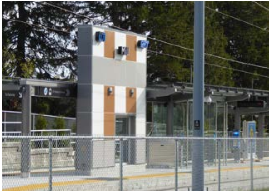
Mill Street ION LRT Station
