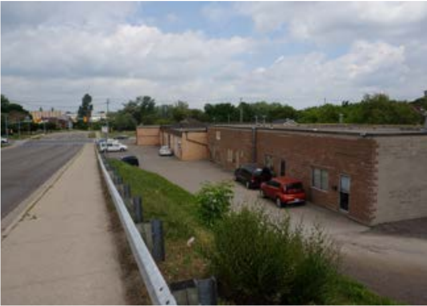
Commercial Uses and grade change at Courtland Avenue and Stirling Avenue
