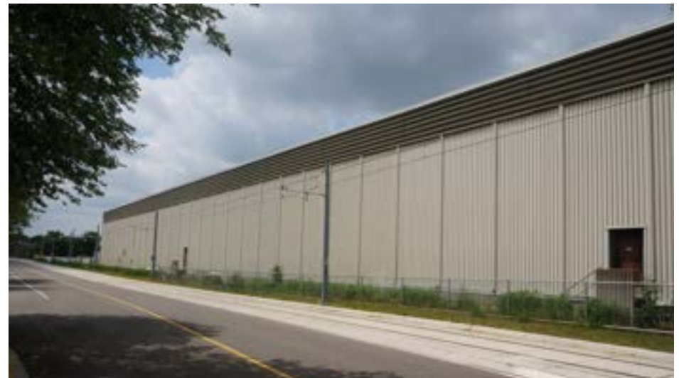
Borden Avenue South Streetscape
