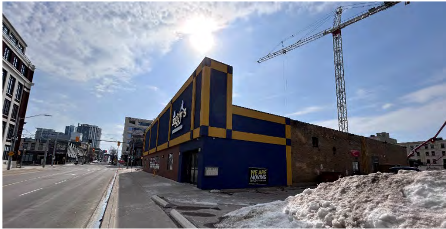
Figure3: view of subject property from King Street (MHBC)
