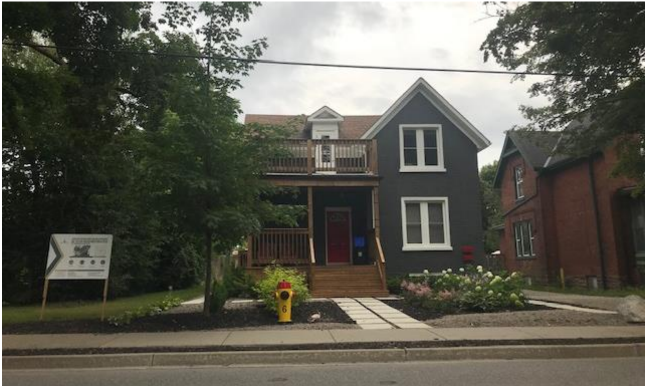
Figure 2 – Existing Duplex Dwelling at 229 Wellington Street North
