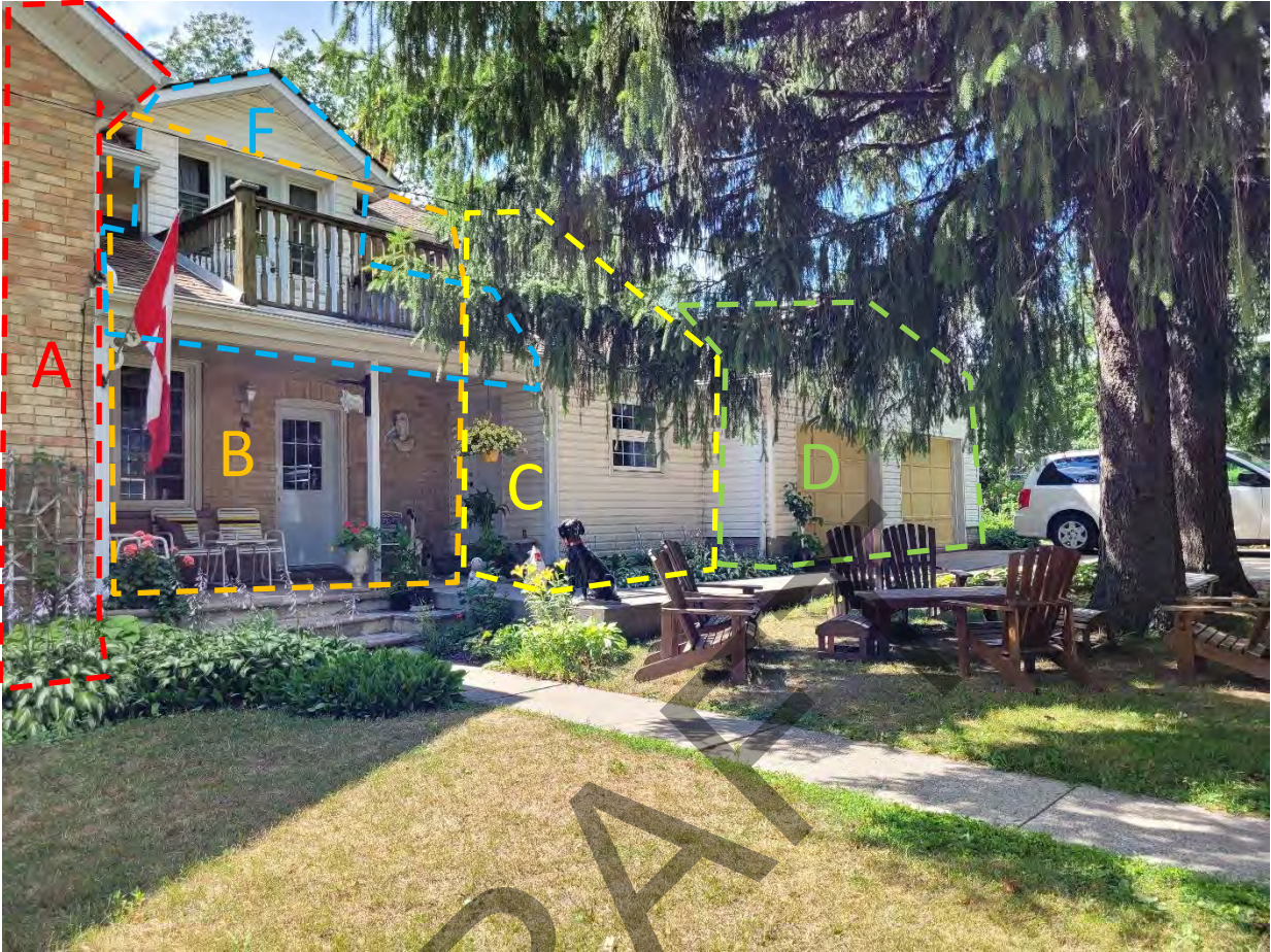
Figure 31: (left) View of east elevation of dwelling (Sections A, B, C, D, and F) (Source: MHBC, 2022)
