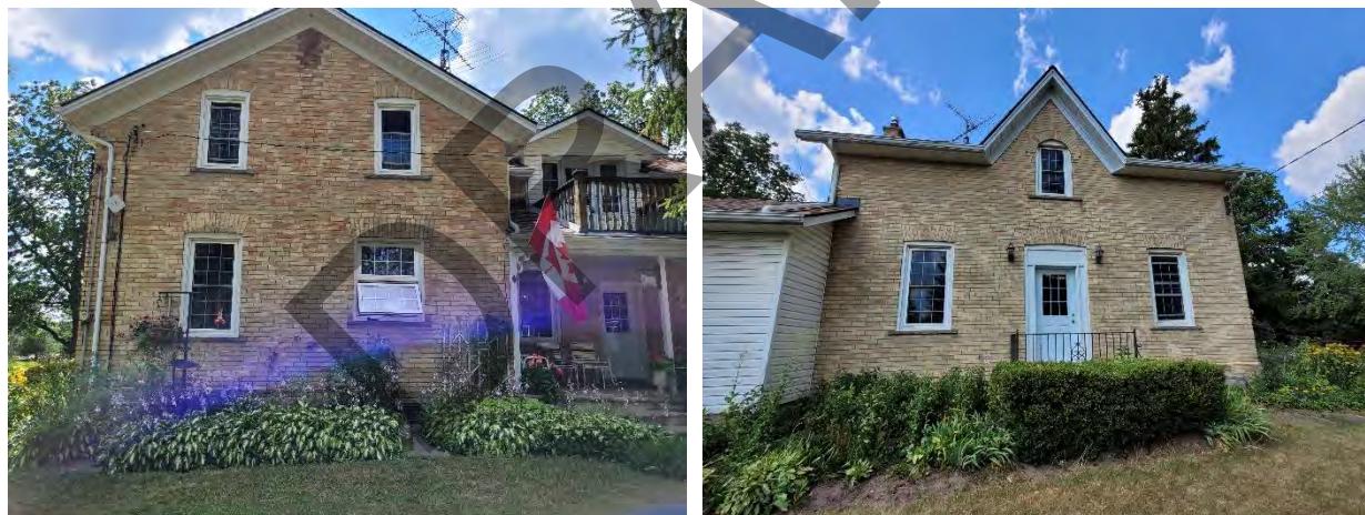
Figures 26 & 27: (left) View of east elevation of Section A, looking west, (right) View of front elevation of Section A, looking north, (Source: MHBC, 2022)
