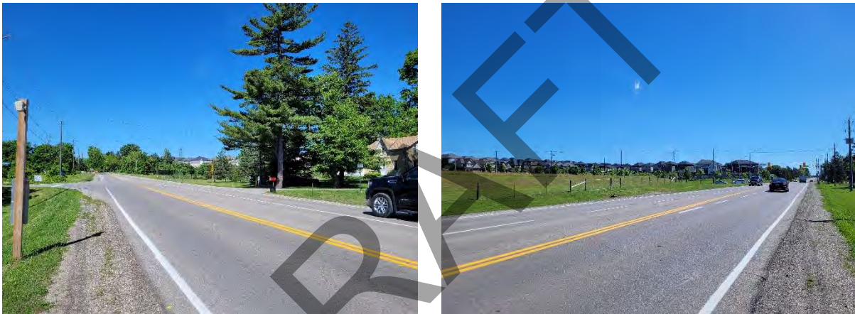
Figures 20 & 21: (left) View of New Dundee Road looking west, (right) View of New Dundee Road looking east towards Robert Ferrie Drive. (Source: MHBC, 2022)
